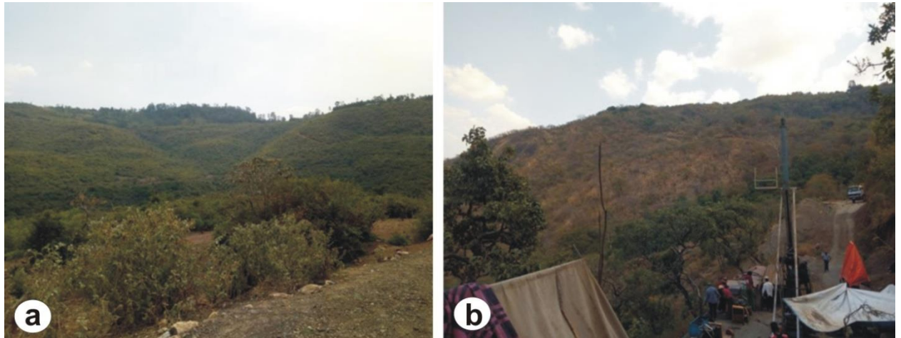
Plate 3.1 (a) Photographic view near to the tunnel portal (b) Surge shaft slope
