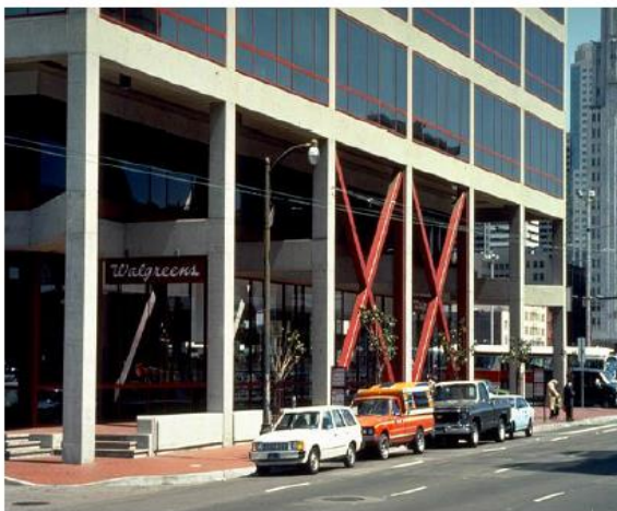
Figure; 2.3 Concentric and Eccentric bracing
