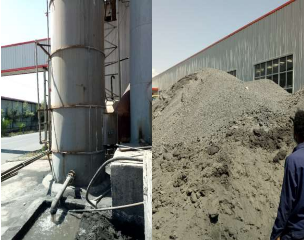
Figure 3-3: Coal ash Collection in Dongfang Spinning Printing and Dying PLC.
