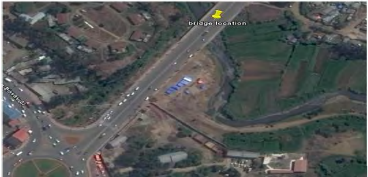
Figure 2. Location of Mekanisa Bridge.
