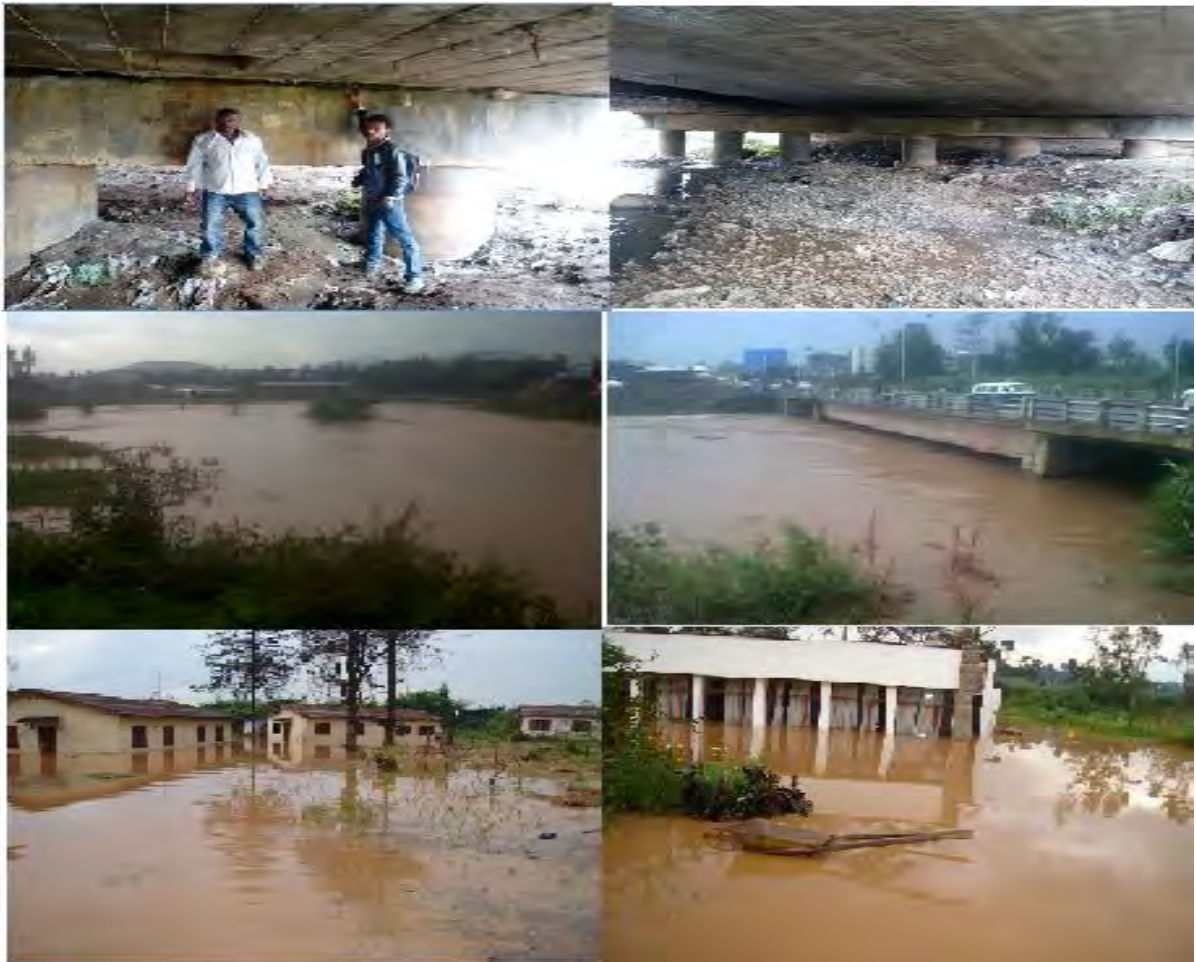
Figure 12. Sediment level under Mekanisa Bridge (Top), flooding just downstream of the Bridge (Middle) and flooding of Office and Dormitories at Mekane Eyesus Seminary compound just upstream of the Bridge (Bottom).
