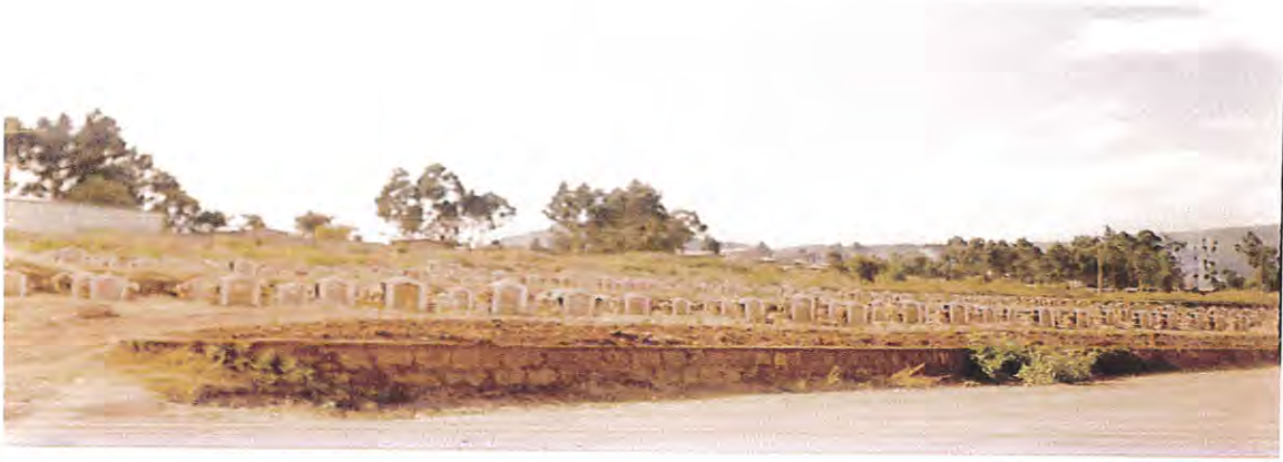
Photo.31: A Block Cemetery that Susceptible for Erosion, Kechene Cemetery (Source: Field Survey, June 2010)
