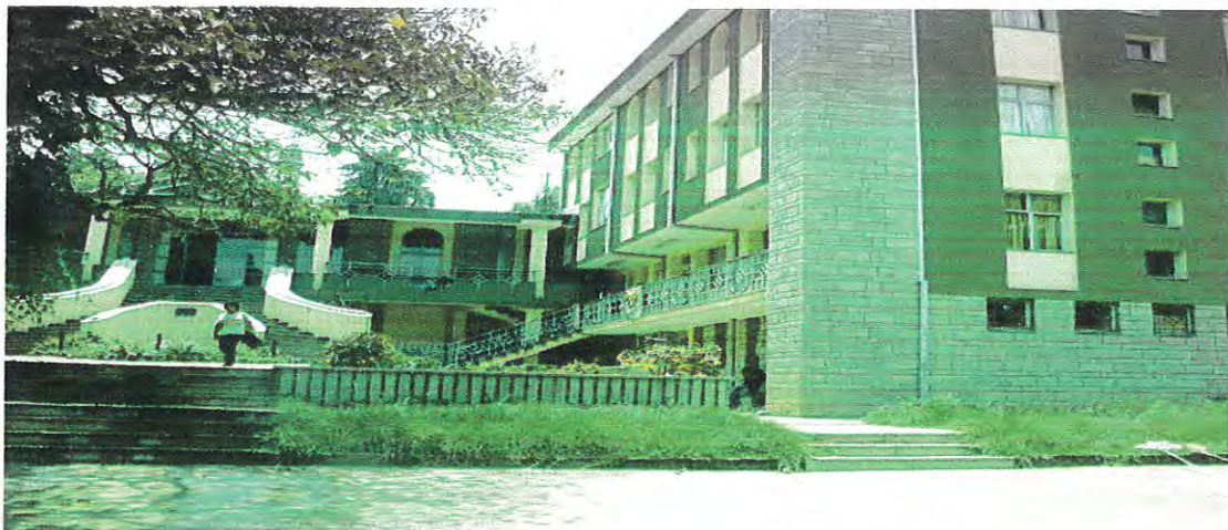
Photo.12: The Multi use Building, Cathedral Menibere Tsebaot Kidist Silase Church (Source: Field Survey, June 2010).
