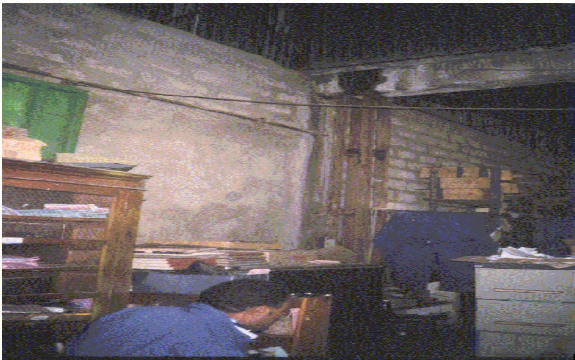
Figure 2.8 a) Shear of tie beam in Addis Ababa city car maintenance hangar [31]
