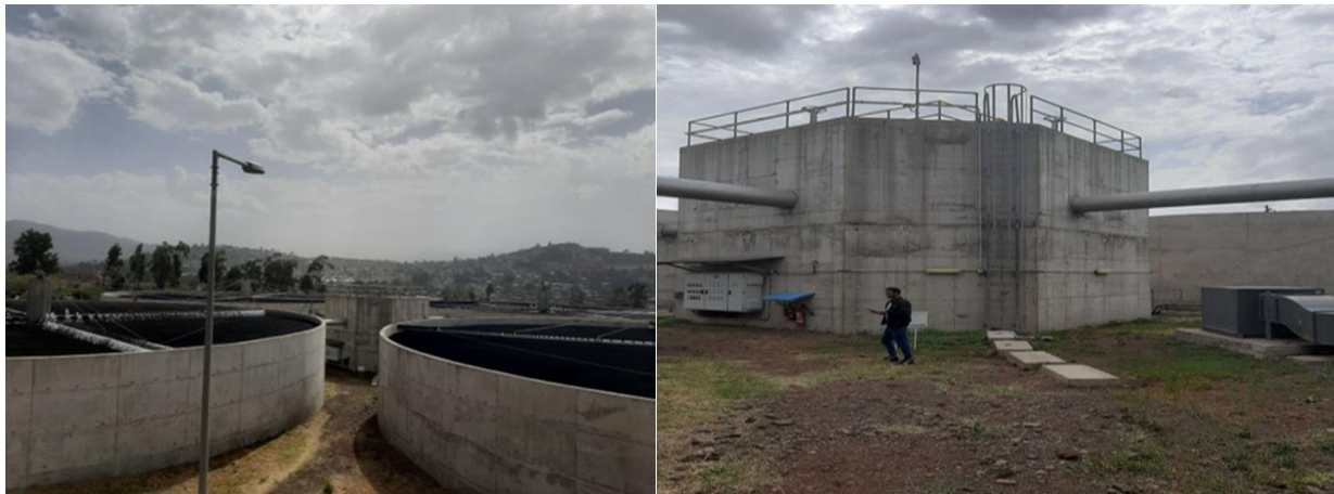
Figure 7 Trickling filter and its distribution system
