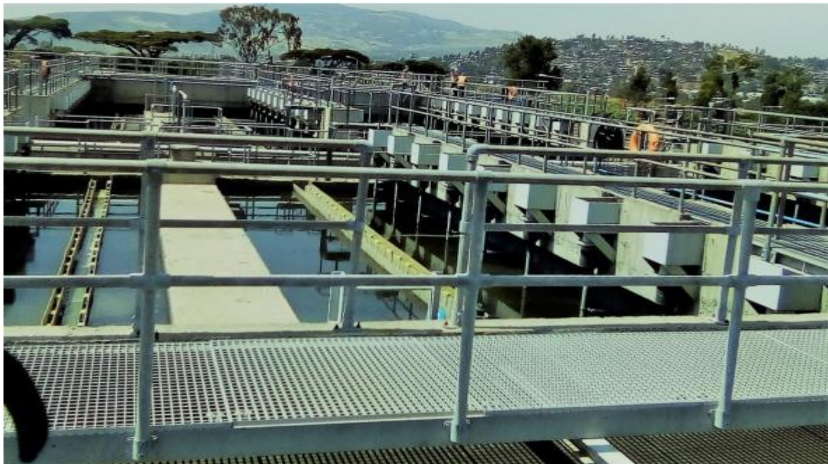
Figure 6 UASB reactor of Kality sewage Treatment Plant (Abewaw, 2021)
