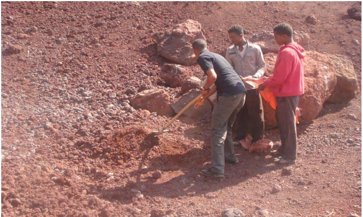
Figure 3.3: Material site for cinder gravel
