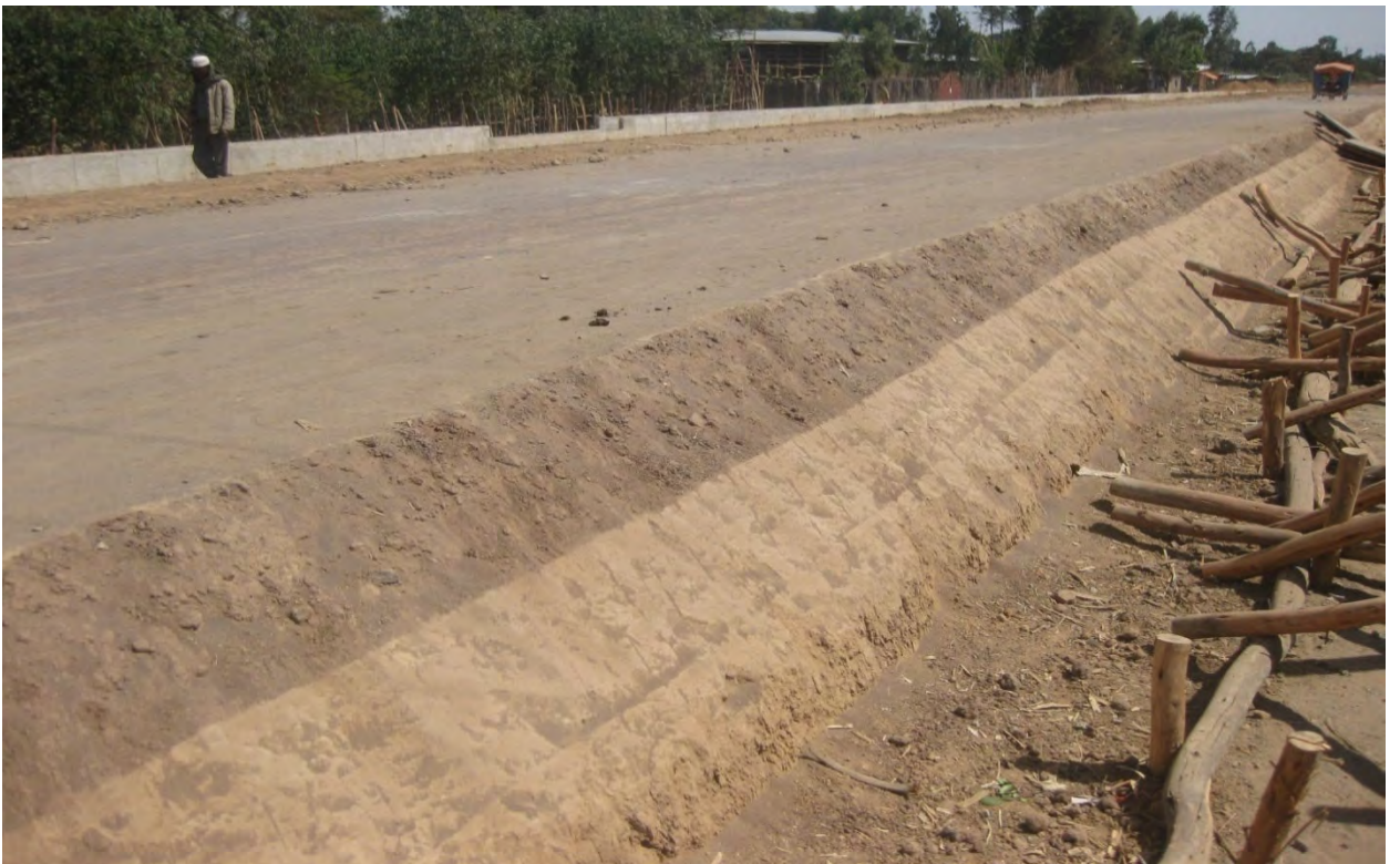
Figure 3.4: Sub-base layer under construction
