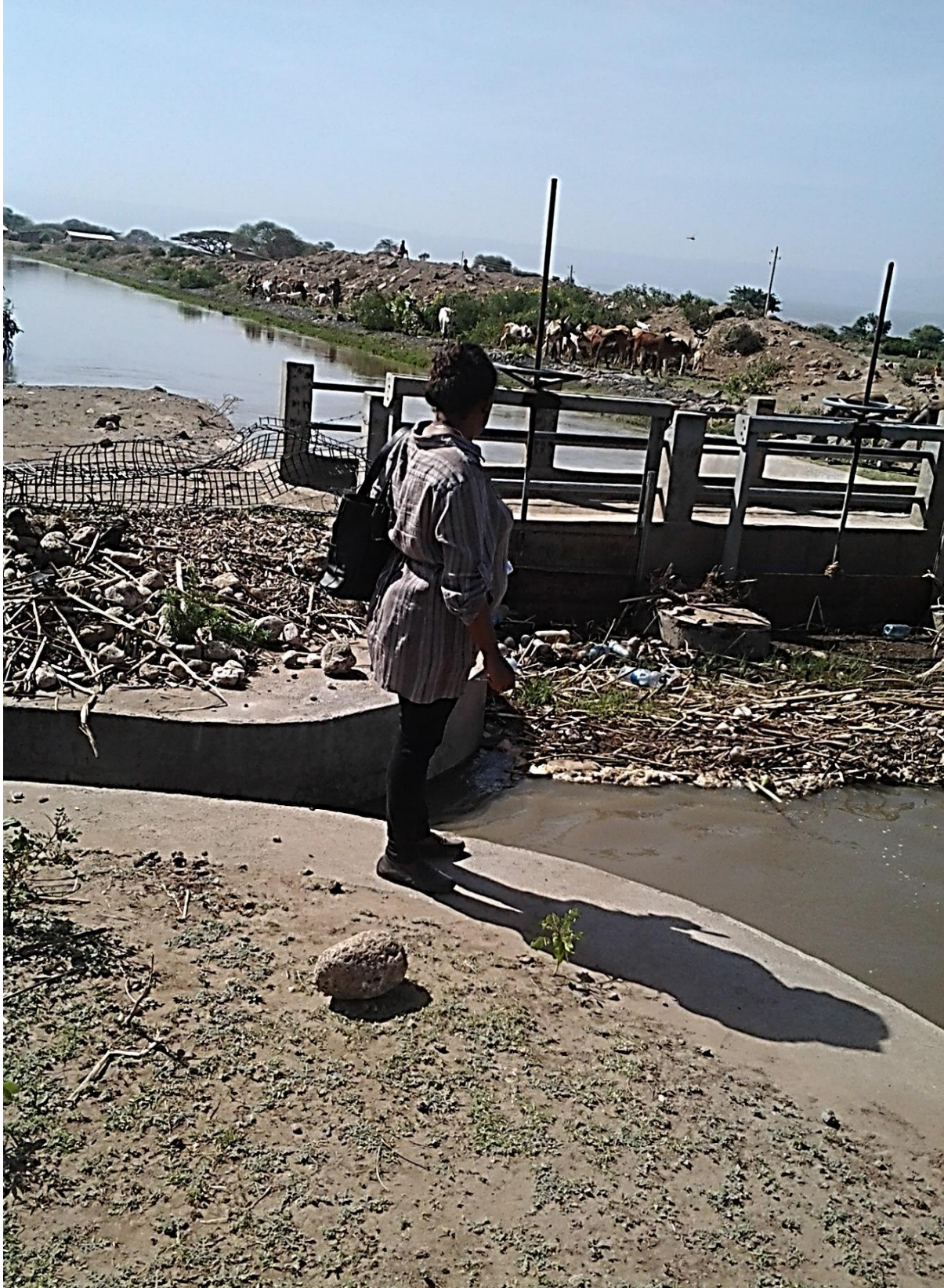
Photo. 4.7. Cross drainage structure
