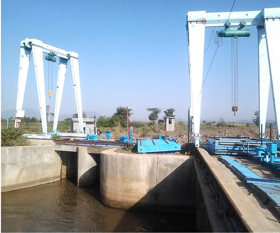
Photo.4.1. Diversion weir Head Regulator
