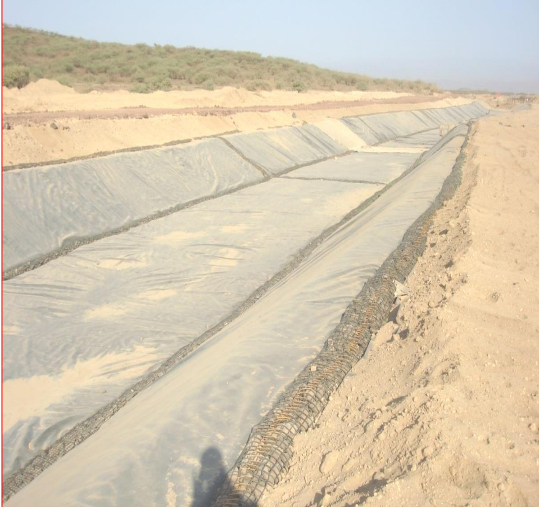
Photo.4.6. Canal lining with geo-membrane
