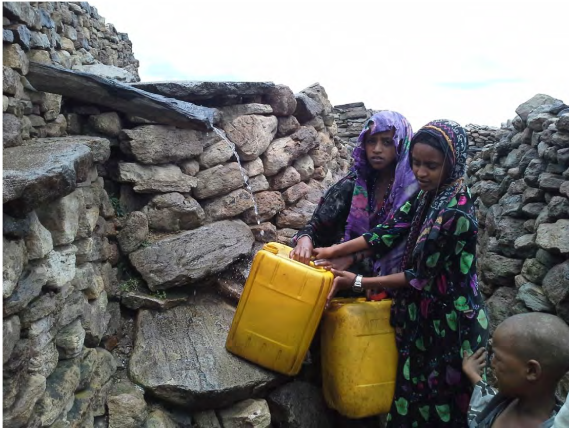
Fig. A32: Potable rain water harvesting from flat roof of house
