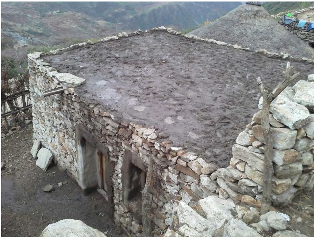
Fig.4:217 mixing of soil with water & ramming with foot.
