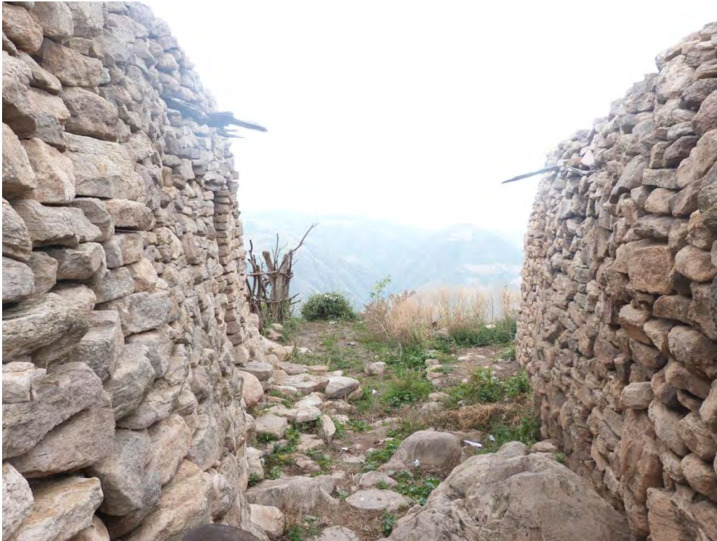
Fig. A52: Service road (toilet and dry waste disposal)
