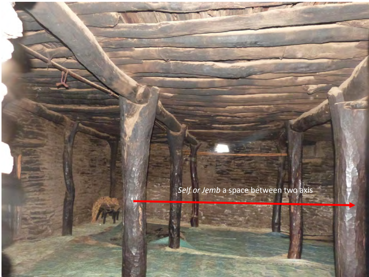
Fig. 4:34 Grid system of column ( Bala ) at dwellings and mosques.
