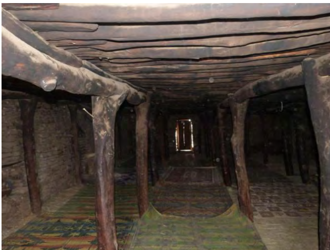
Fig.4.29 interior of Hutuba of Hutuba mosque
