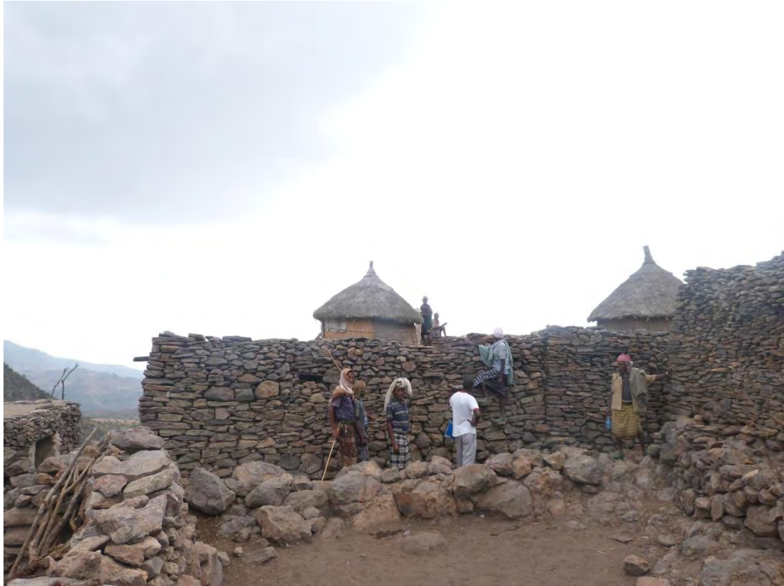
Fig. A56: G+1 house masonry work at Toleha Amba
