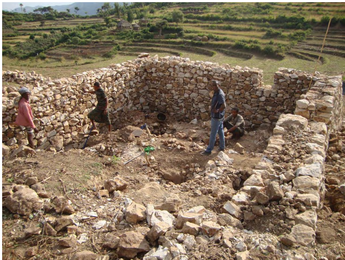
Fig. A37: Masonry work of house
