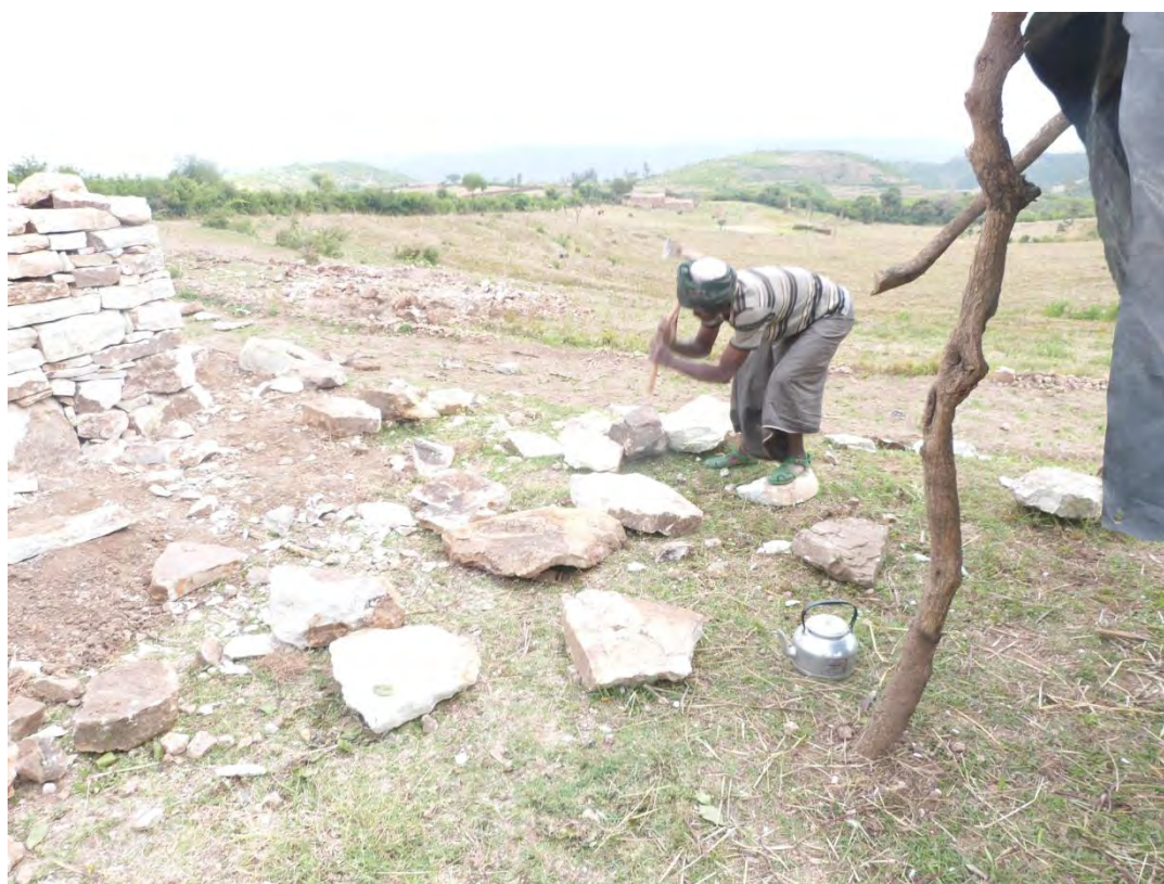
Fig. A39: Cutting and shaping of stone for house
