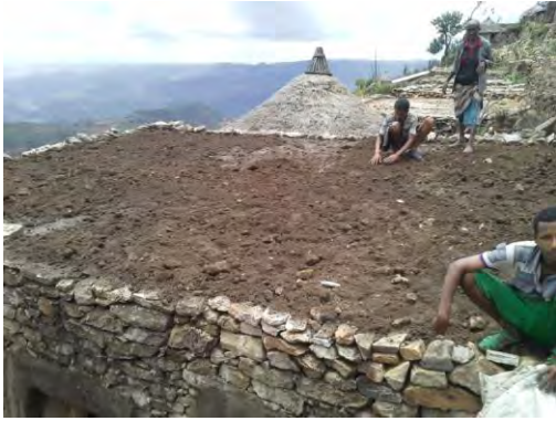
Fig.4:218 adding of 2-3cm thick gravel to the rammed roof slab.
