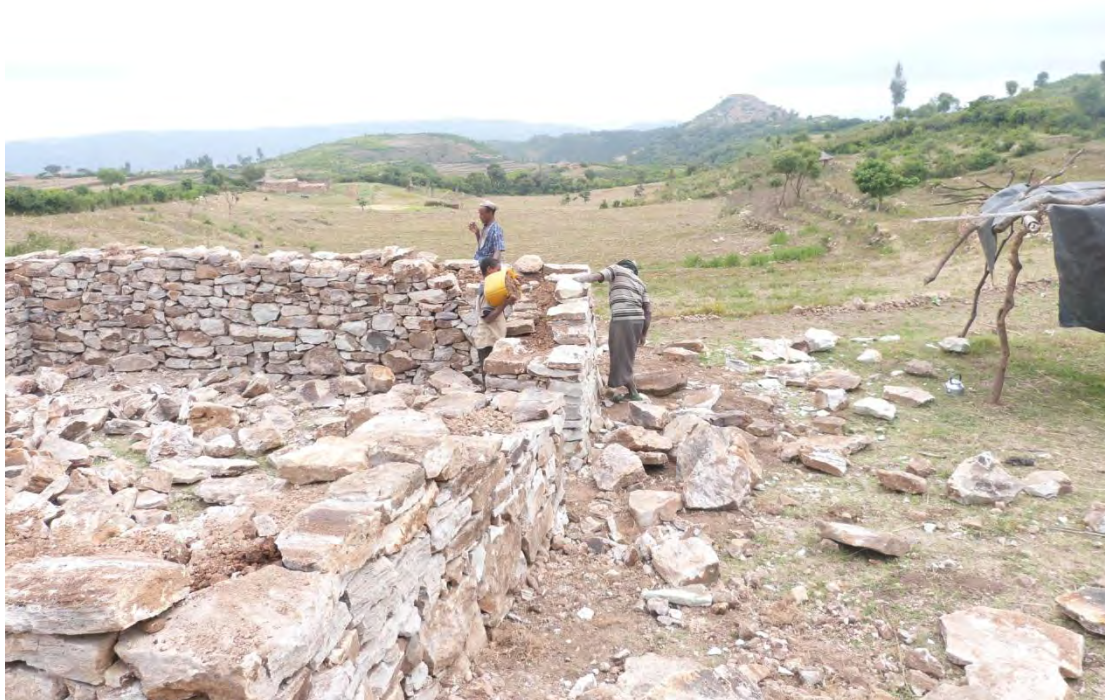
Fig. A38: Masonry work of house
