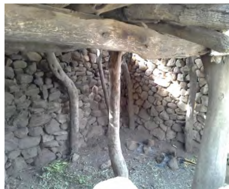
Fig. A2-14 Columns main beam at Wodaja Amba
