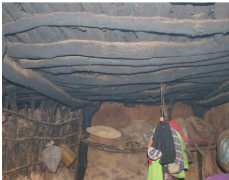
Fig.4:73 Storage at Women's
