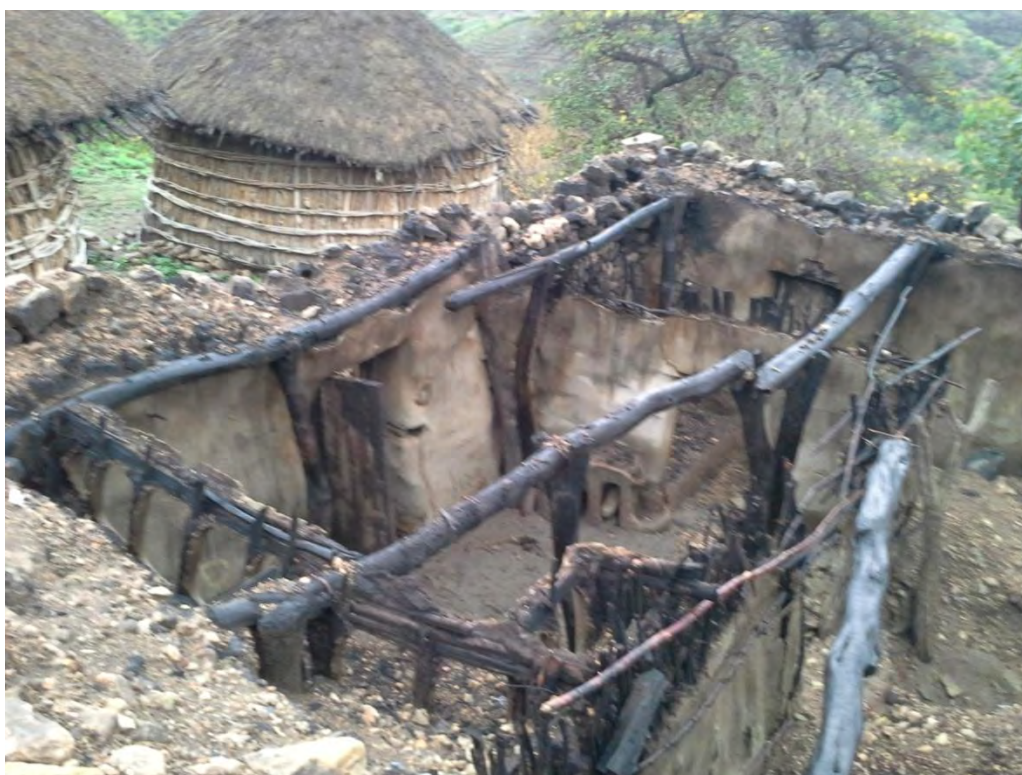
Fig. A80: Demolished house for the ned of columns & other wooden elements
