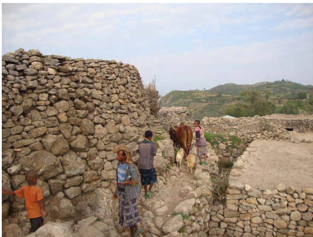
Fig. A83: Activity on main access road
