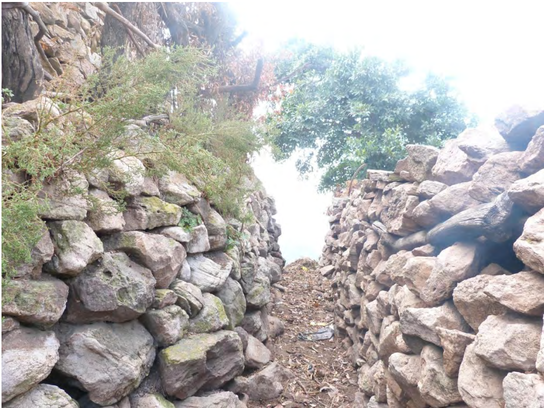
Fig. A53: Service road (toilet and dry waste disposal)
