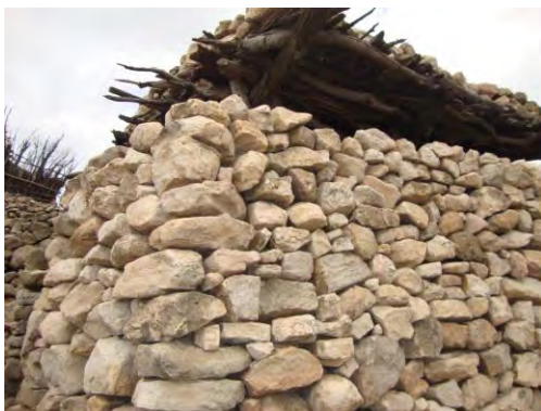
Fig. A2-13 Ventilation at wall of Wodaja Amba
