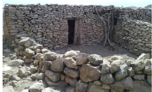
Fig.4:156 Front elevation & front yard
