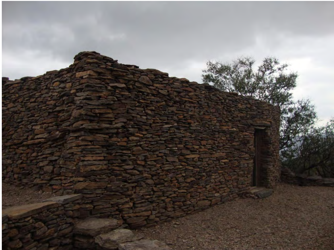
Fig. A55: Refined masonry works at Toleha Amba
