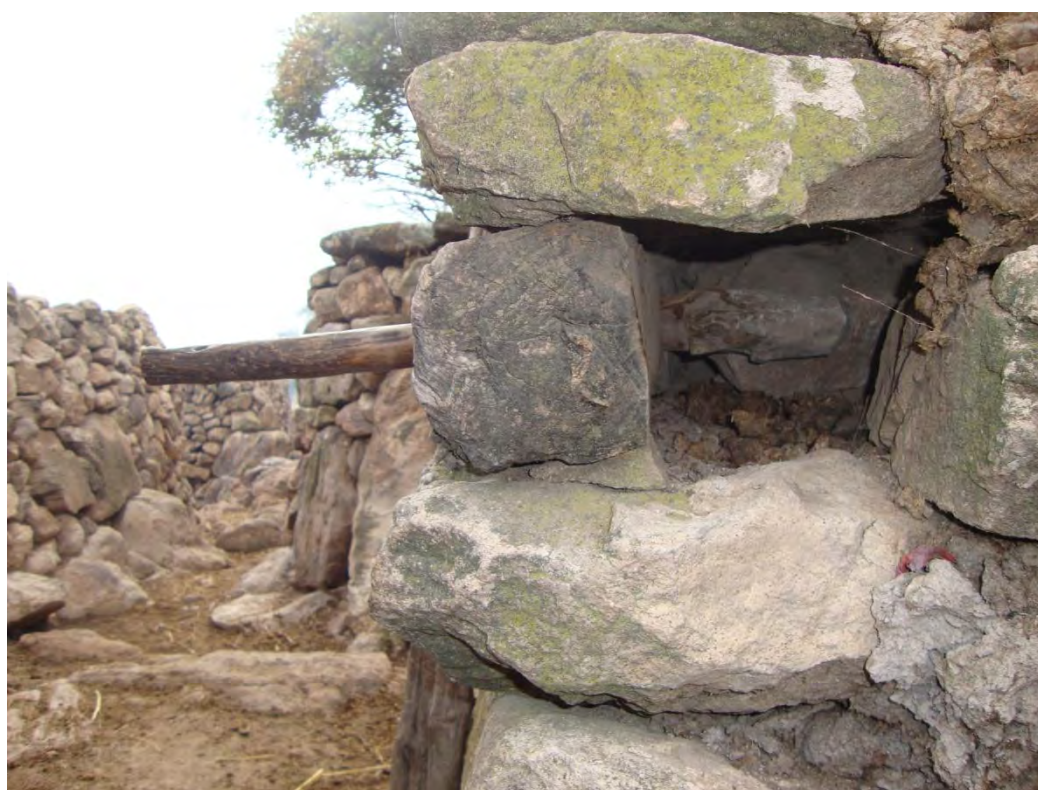
Fig. A63: Door lock system at main gate
