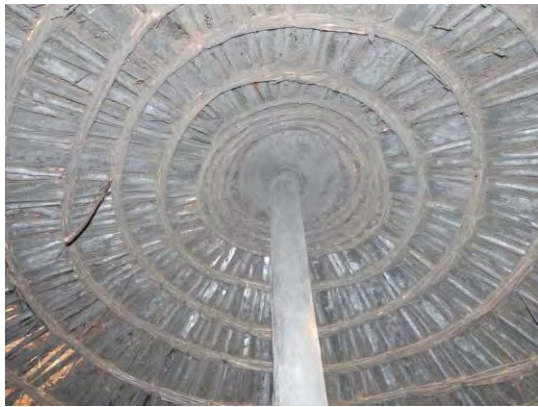
Fig.4:305 internal roof detail of thatched roof house
