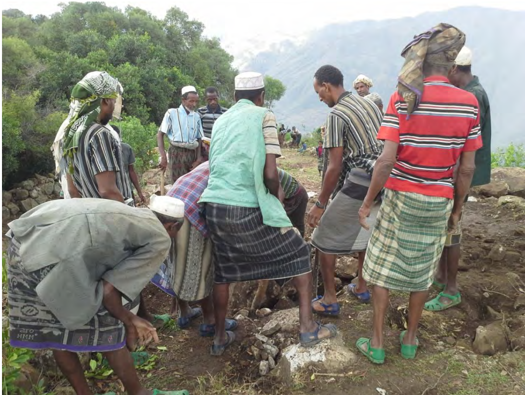
Fig. A49: Access road construction
