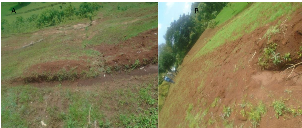
Figure 11; Failed soil bund structure filled by soil sediment
