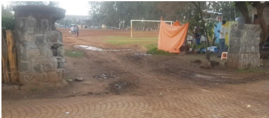
Figure 4.79 Main gate _ Source: Field Survey, 2023
