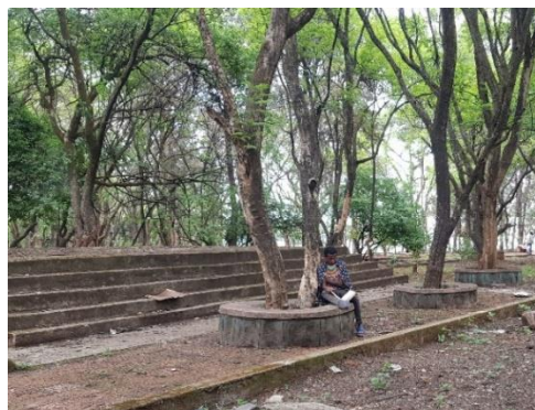
Figure 4.24 Condition of seating
