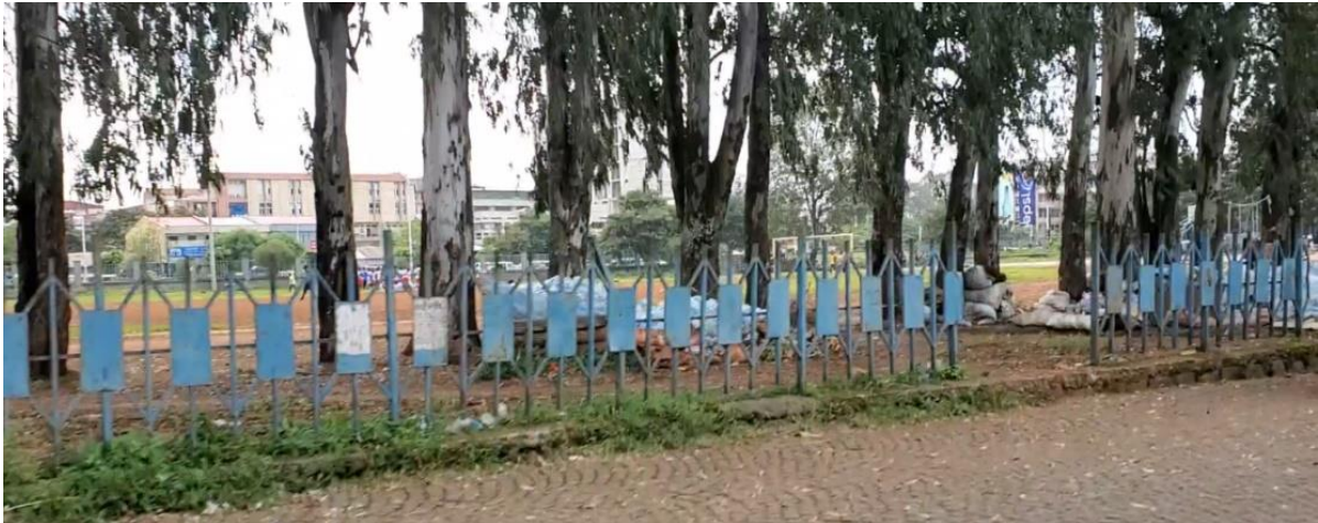
Figure 4.72 Steel frame fence transparency
