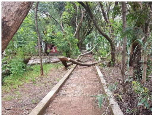
Figure 4.45 Tree fall in to walk way
