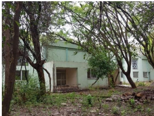
Figure 4.36 Library building cover with construction material
