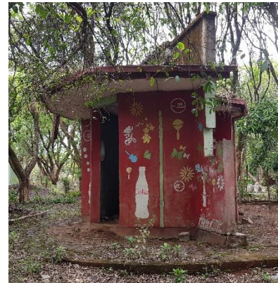
Figure 4.13 Public toilet with painting wall
