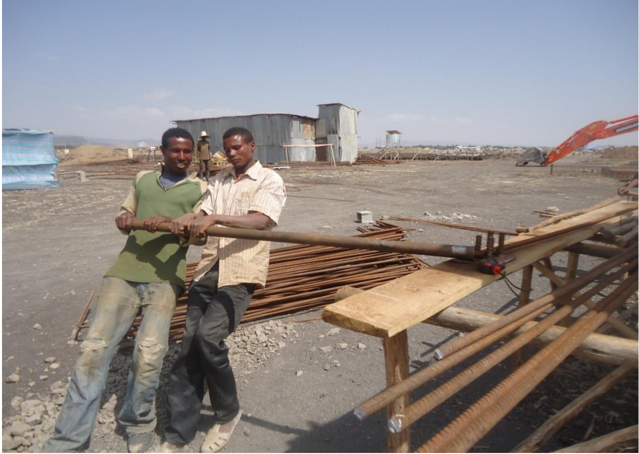
Figure 4.16.Site bending of reinforcement bar in Bole Arabsa site
