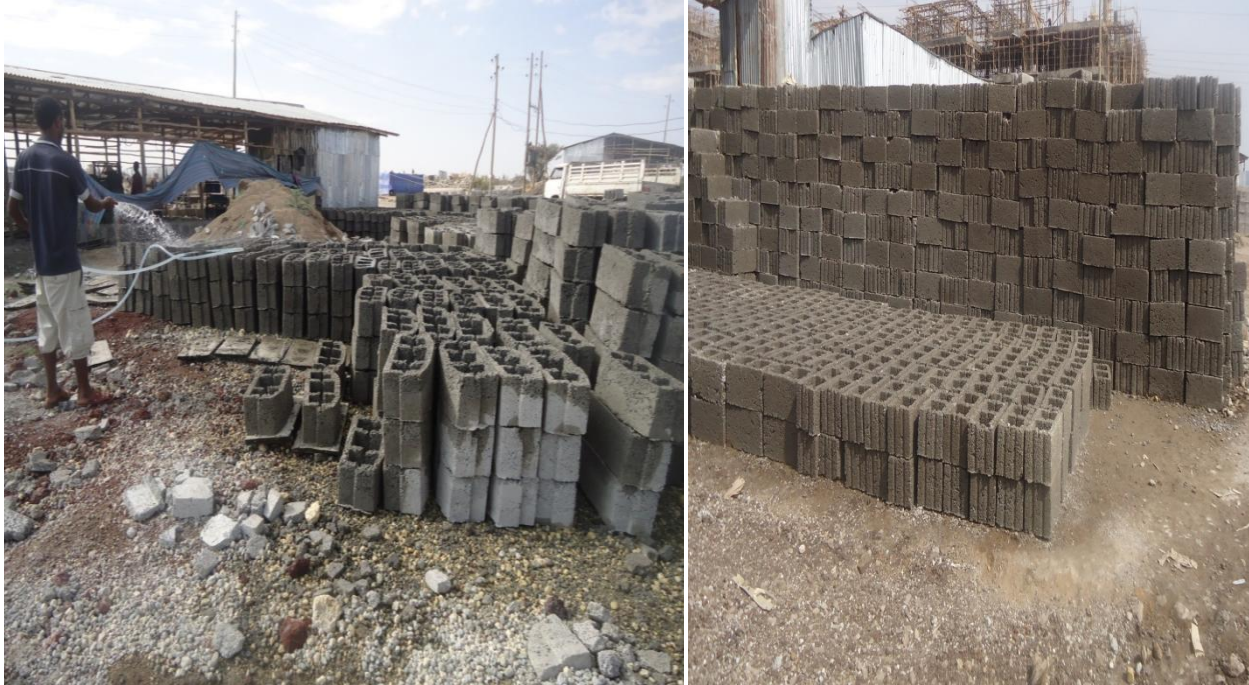
Figure 4.21 Curing of hollow concrete block in Bole Arabsa site site
