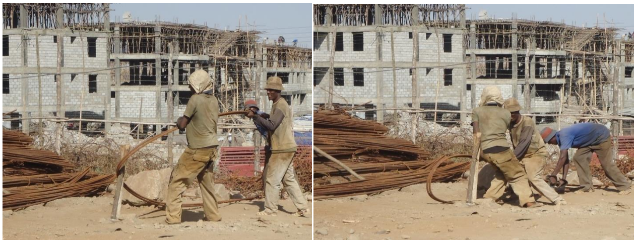
Fig 4.14 bending of reinforcement bar in Yeka Abado site
