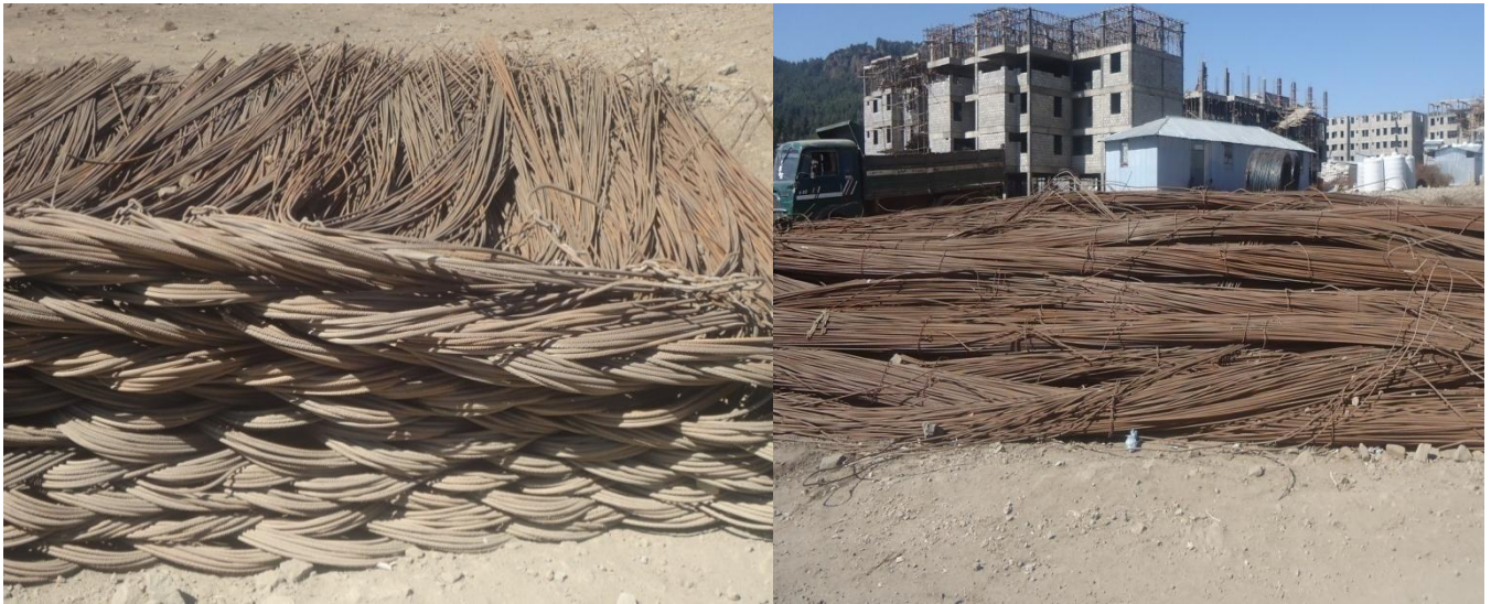
Figure 4.13 Kifle ketema rebar storage in yeka abado site
