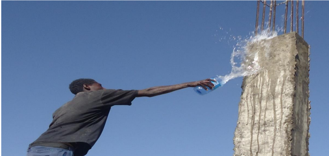
Fig 4.10 curing of concrete in Bole Arabsa site
