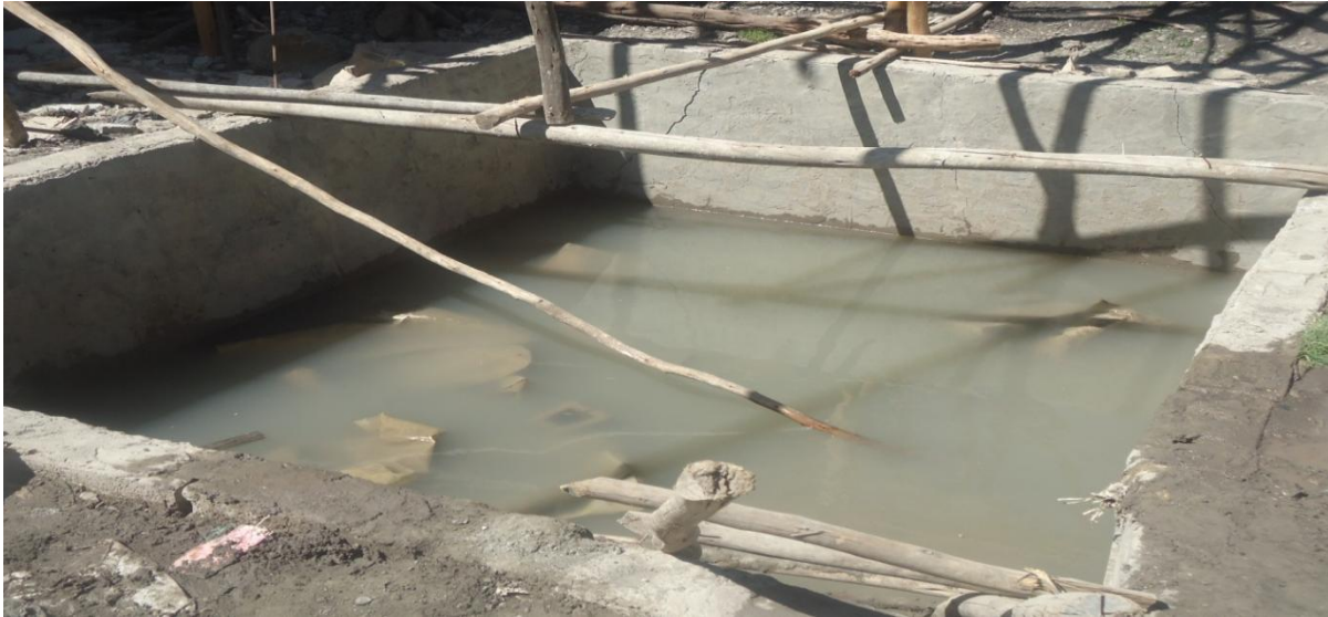
Figure 4.6 water tank in Kolfe keranyo site
