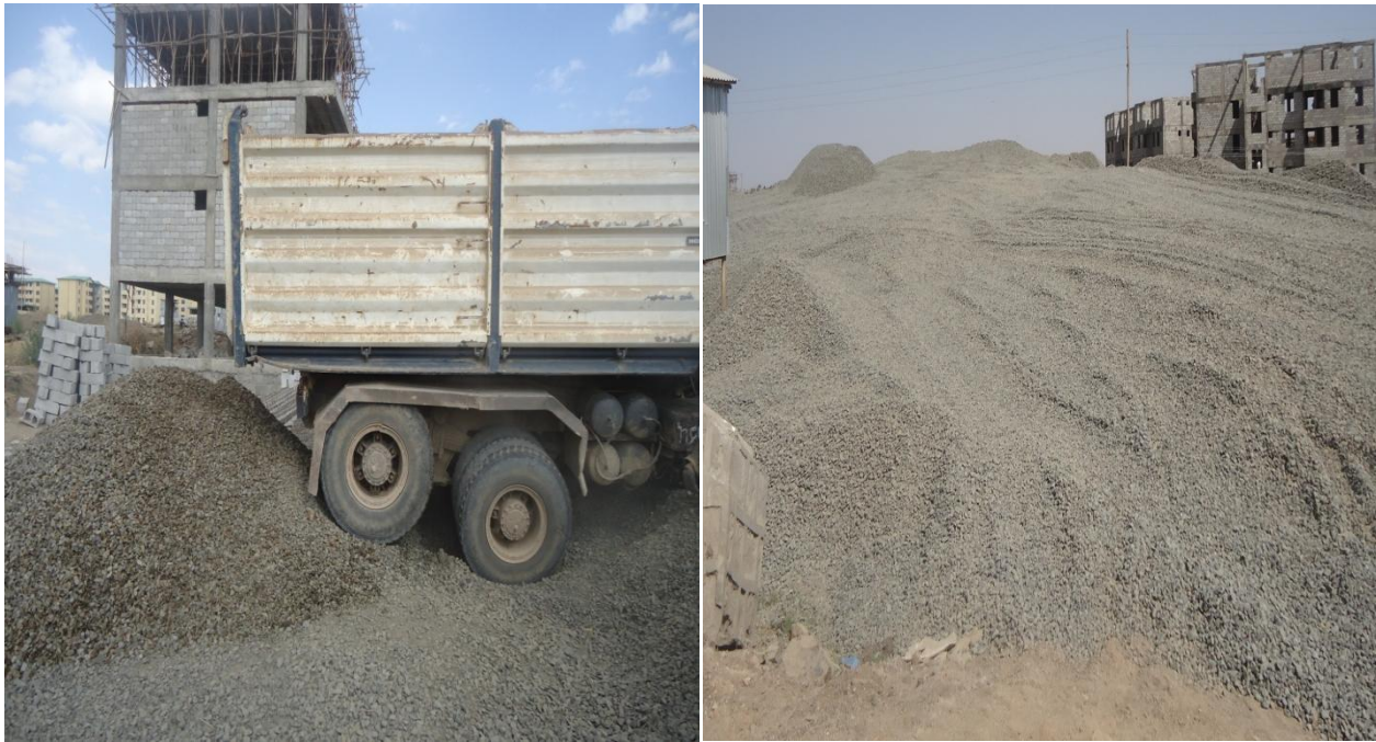
Fig 4.3 dump truck moving on the coarse aggregate in Ayat site and Yeka Abado
