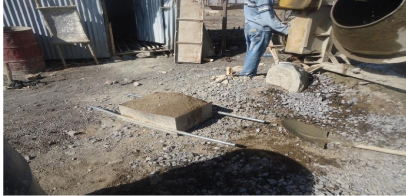
Fig 4.7 batching of fine aggregate in bole Arabsa site
