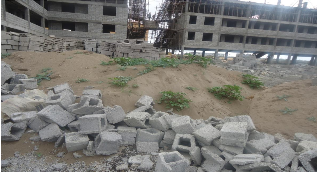
Fig 4.4. Handling of fine aggregate in Ayat III site
