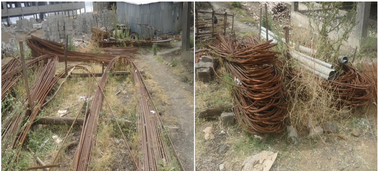
Fig 4.15 stacking of rebar in construction site in Ayat site
