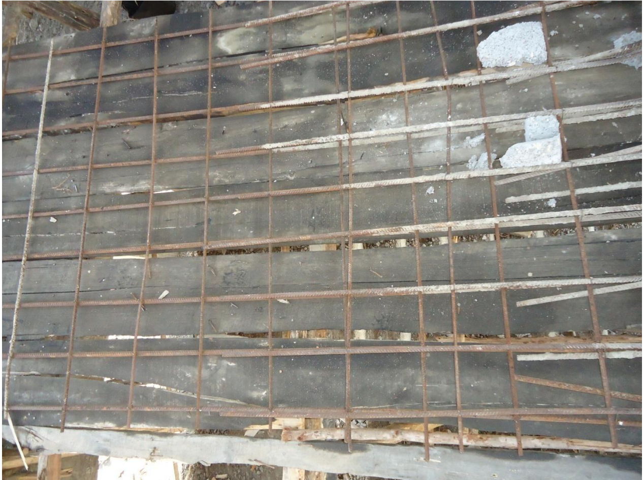
Figure 4.17. Reinforcement bar ready for concreting in Bole Arabsa site
