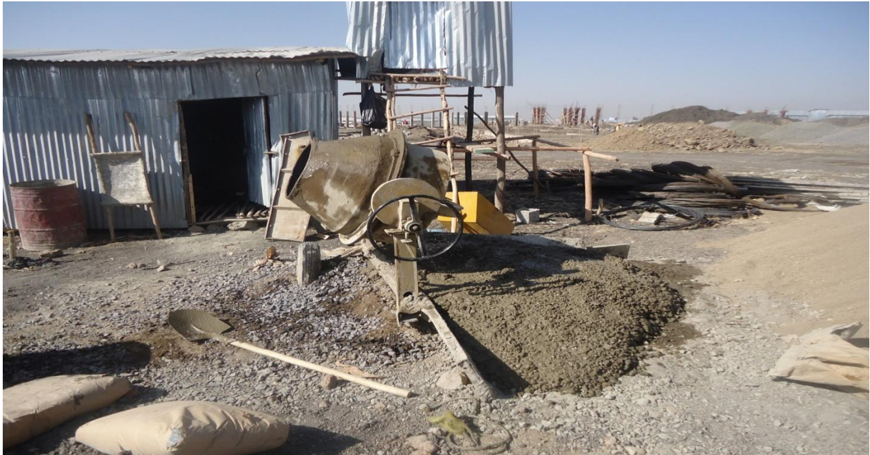
Fig 4.8 discharged fresh concrete on the site in Bole Arabsa site
