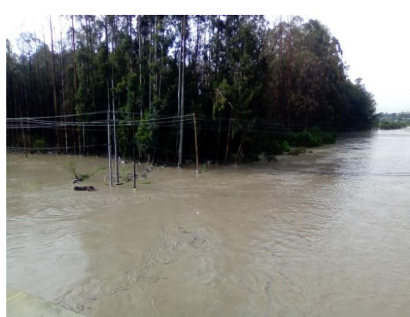
f. Flood overtopping during 2020 season
