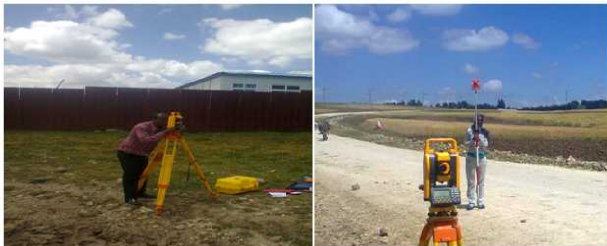
Figure 3.2. Gathering of Gravel Loss Data
