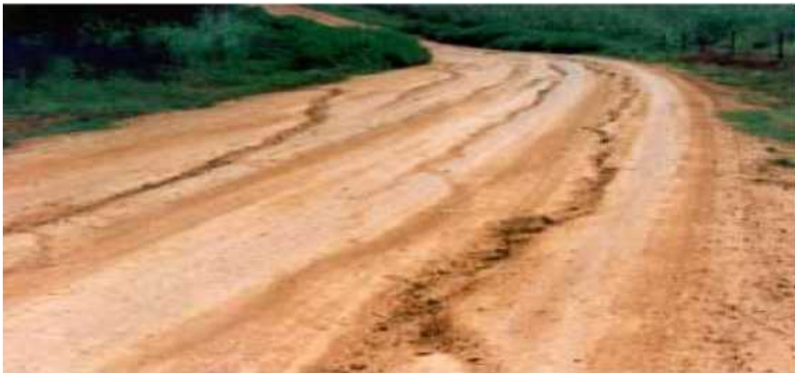
Figure 2.6: longitudinal erosion
