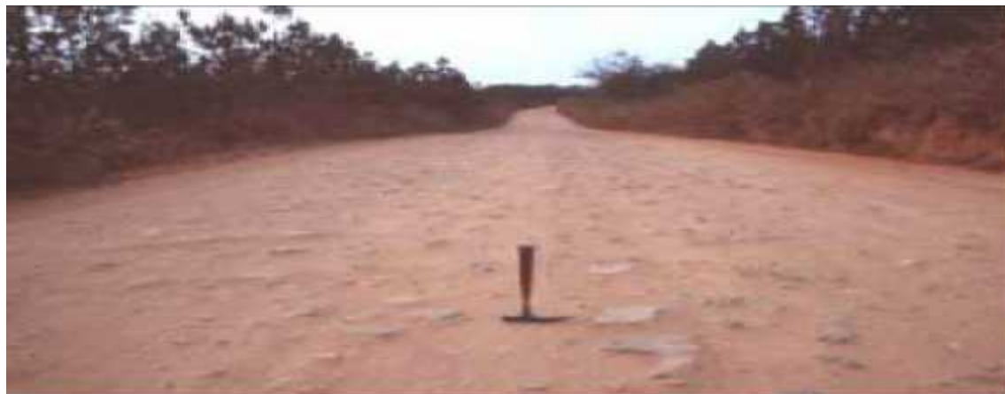
Figure 2.8: Severe embedment of stones
