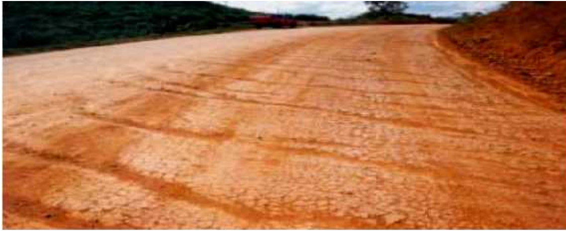
Figure 2.5: Transversal erosion
