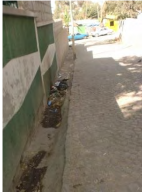
Figure 6.16: Solid wastes on drainage system
