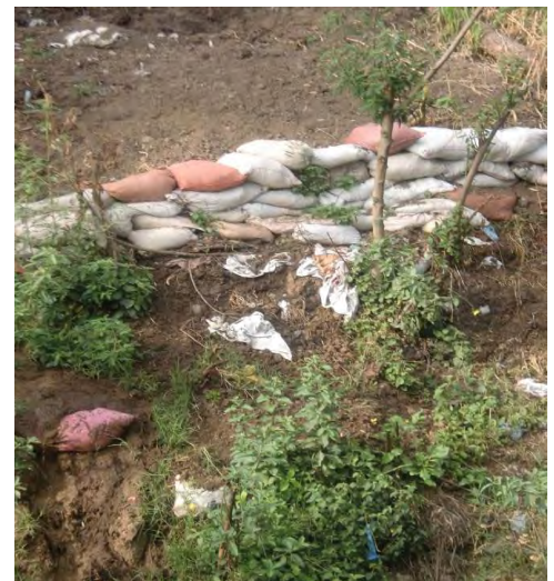
Figure 5.5: put soil in sack and place it along the river.
