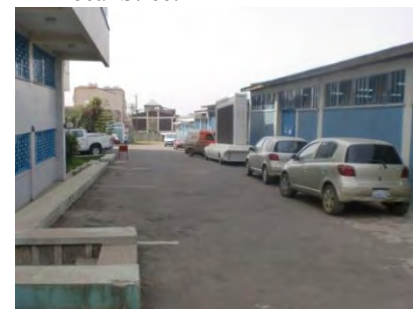
Figure: 6.21f parking lot in Alemayehu building
