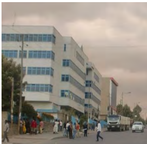
Figure 6.27: Lack of green roof, Alemayhu Building
