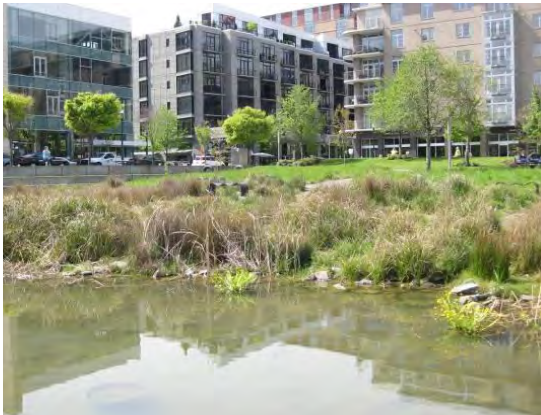
Figure 3.7: Detention pond (wet) in Tanner Springs Park, Portland, Oregon, USA
