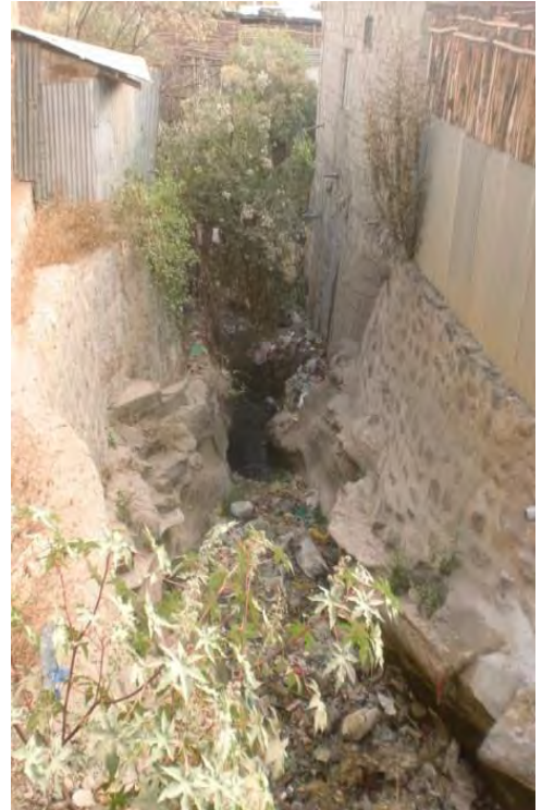
Figure 5.4: Digging deep the bottom surface of the water
