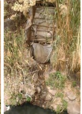
Figure 6.19: Toilet directly linked with Finicha River
