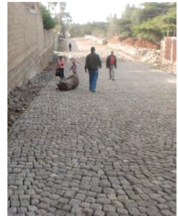
Figure 6.35a: local road Paved with cobble stone
