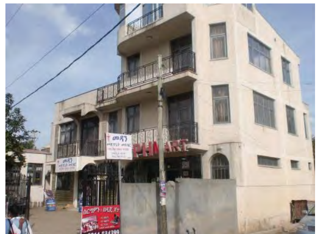
Figure 6.28: Surface of the mixed use compound paved with concrete
