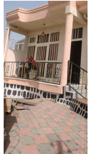
Figure 6.26: Surface of residential compound paved with tiles
