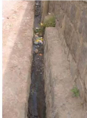
Figure 6.17: Liquid wastes discharged through Open-Ditch
