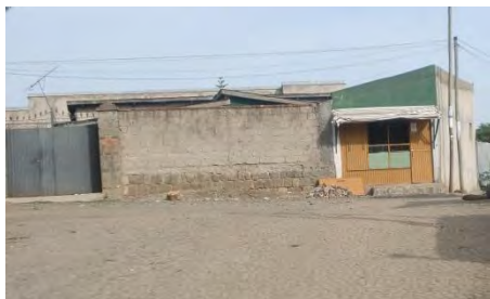
Figure 6.23: Absence of green roof
