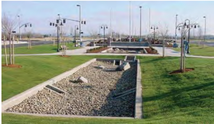
Figure 3.13: Sand filters can be installed above ground.
