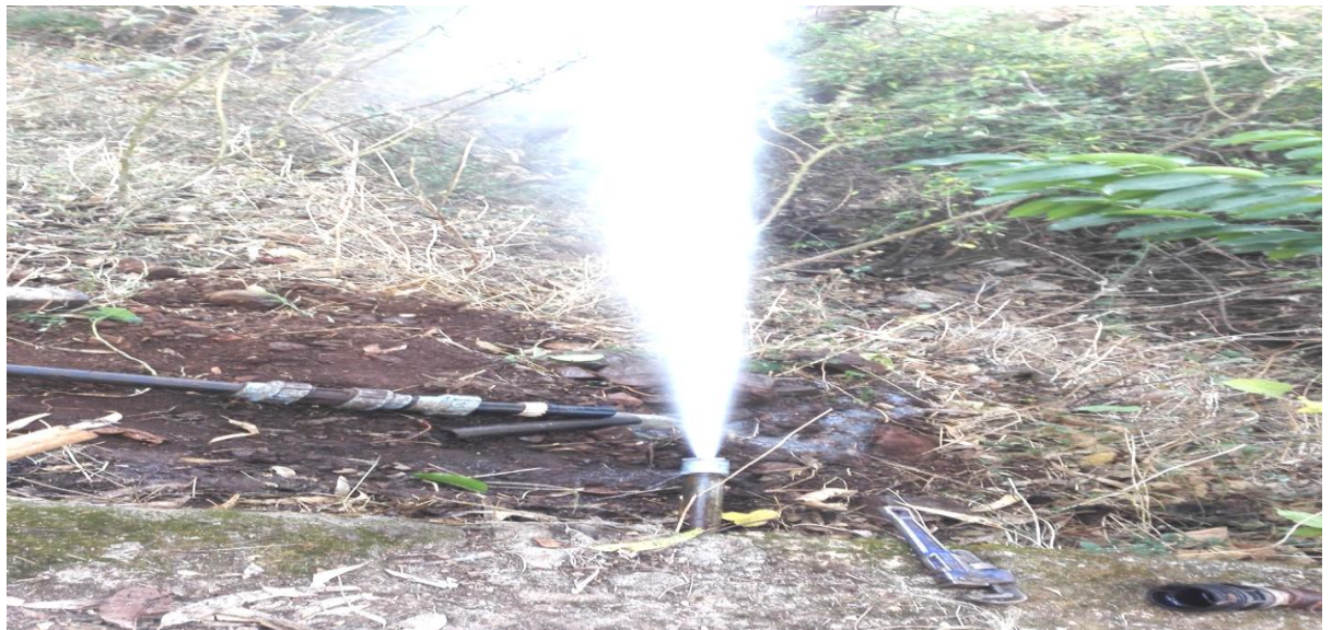
Figure.6. Pressure Measurement at different location
