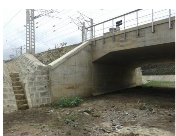
Figure 3e: Left Abutment
