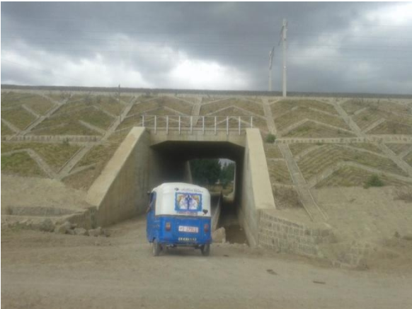
Figure 4b: Upstream view
