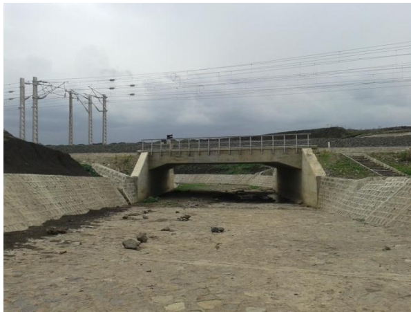
Figure 3b: Upstream View
