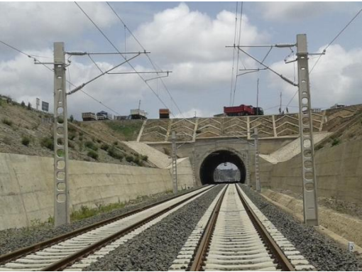
Figure 1d: Upstream View
