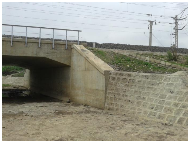
Figure 3d: Right Abutment
