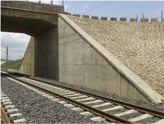
Figure 5d: Right Abutment
