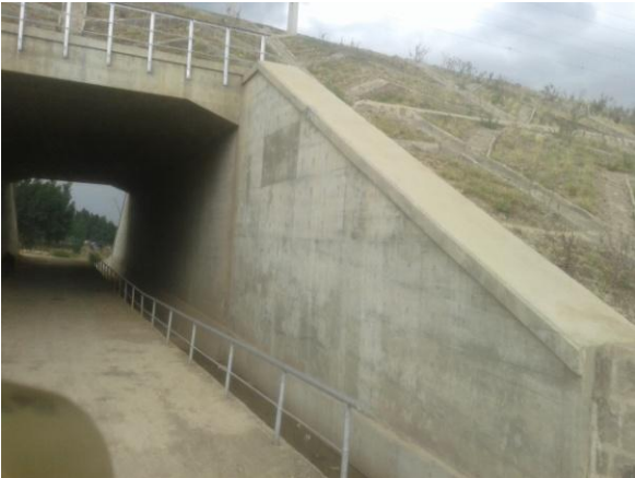
Figure 4d: Right Abutment
