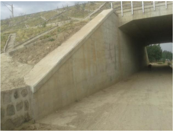
Figure 4e: Left Abutment
