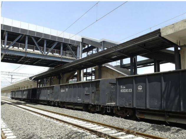
Figure 2d: Right Stair View
