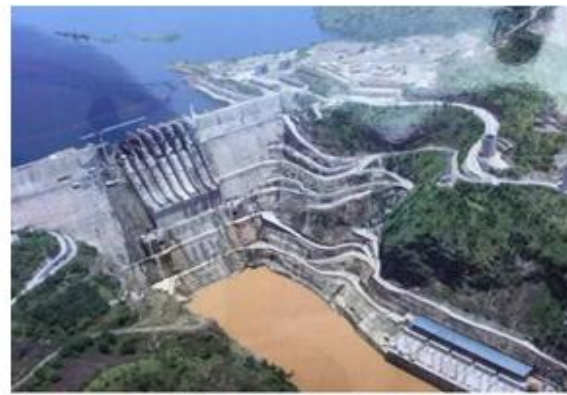
View of the dam from downstream
