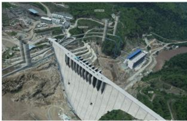
upstream view of the dam
