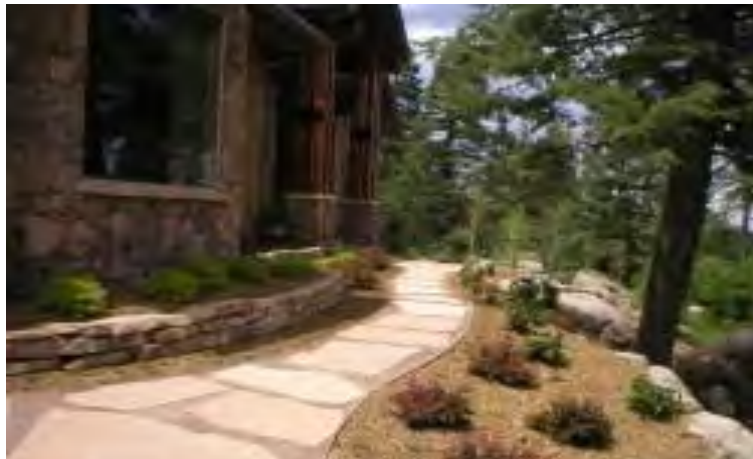
Fig 2. 4 Flagstone pathways with soil cement between joints (Source: Blue fox farm)
