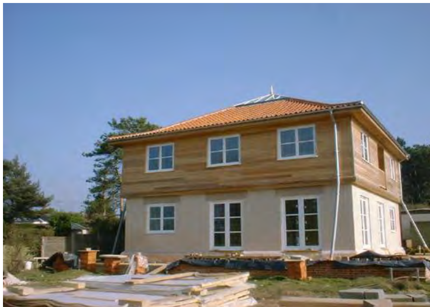
Fig 2.2 Rammed Earth House under construction, (Source: Review of Rammed Earth construction)
