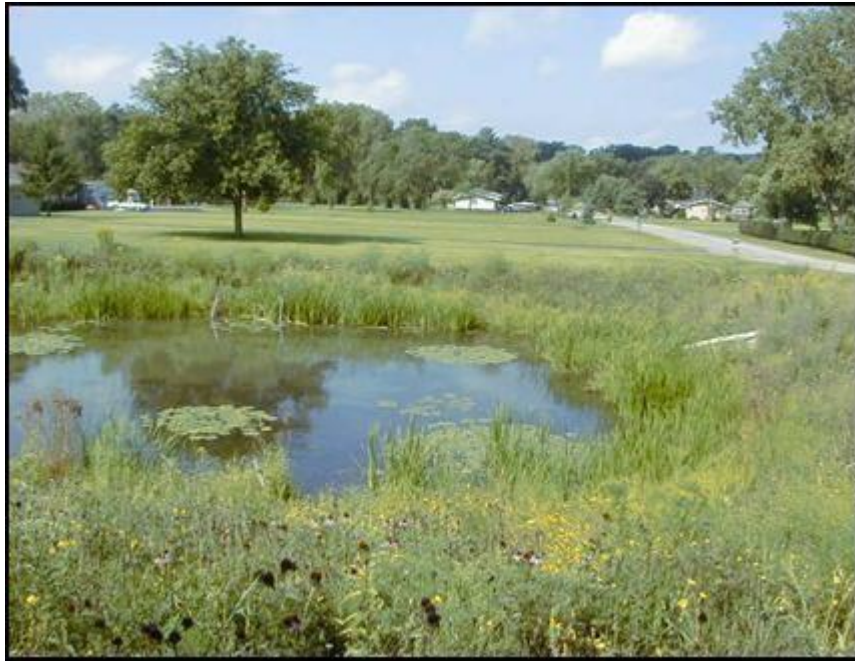
Figure 2. 7: Constructed wetland for storm water management
