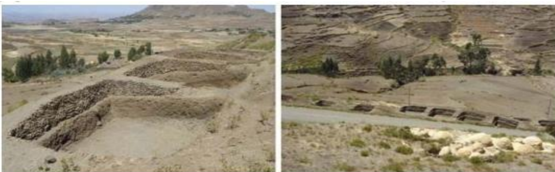
Figure 2. 16: Percolation ponds to collect water from road, Zata area, Southern Tigray , 2018
