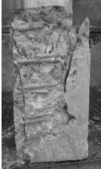
Figure 4-15 Typical Failure of Rectangular Reinforced Concrete Specimen
