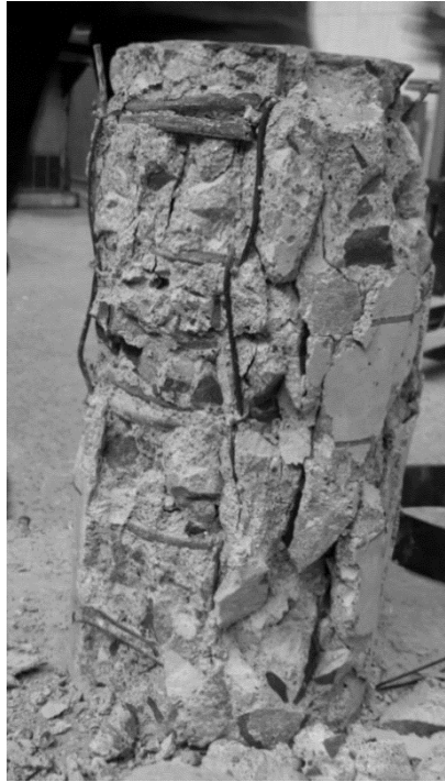
Figure 4-4 Typical Failure of Circular Reinforced Concrete Specimen A
