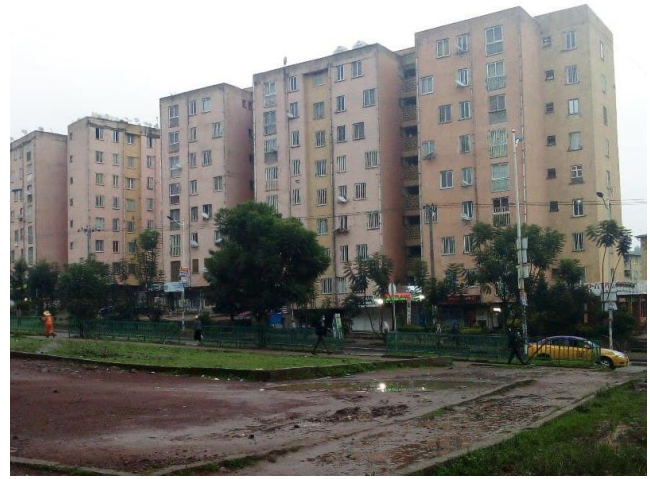
photo 4:G+7 blocks in G7 area
