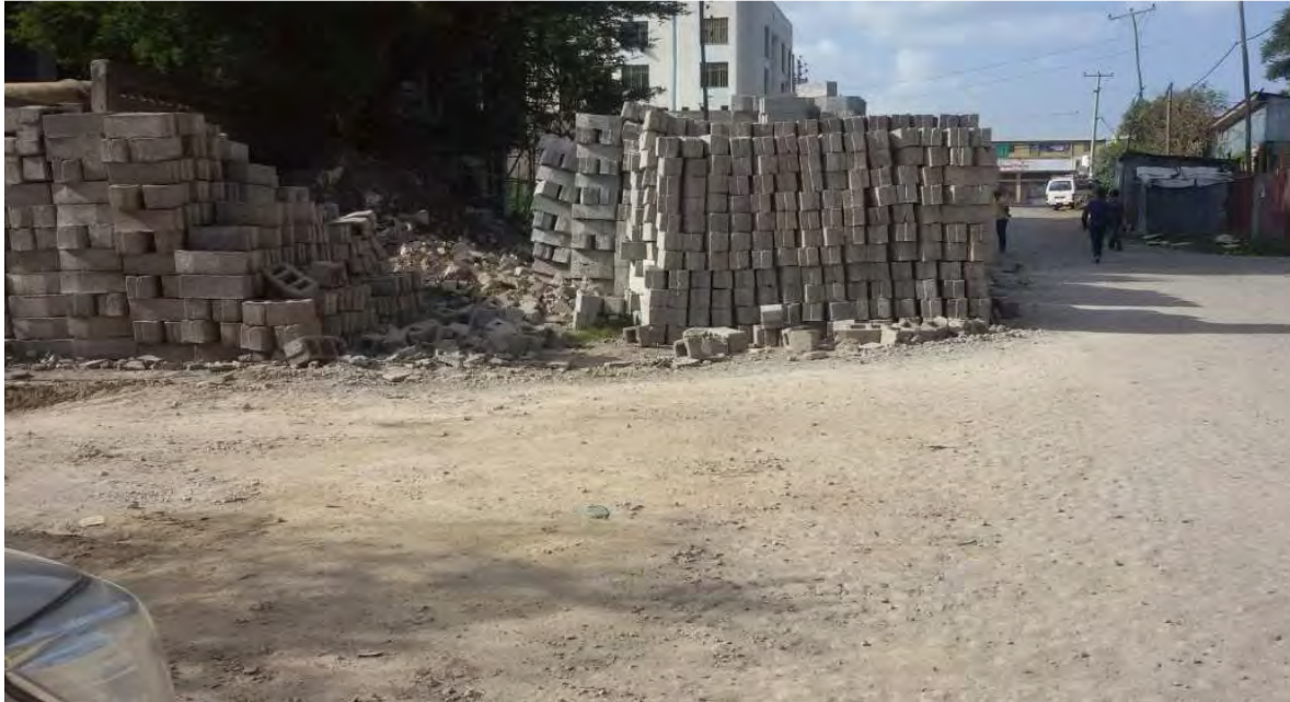
Figure 4.13 HCB stored outside the site
