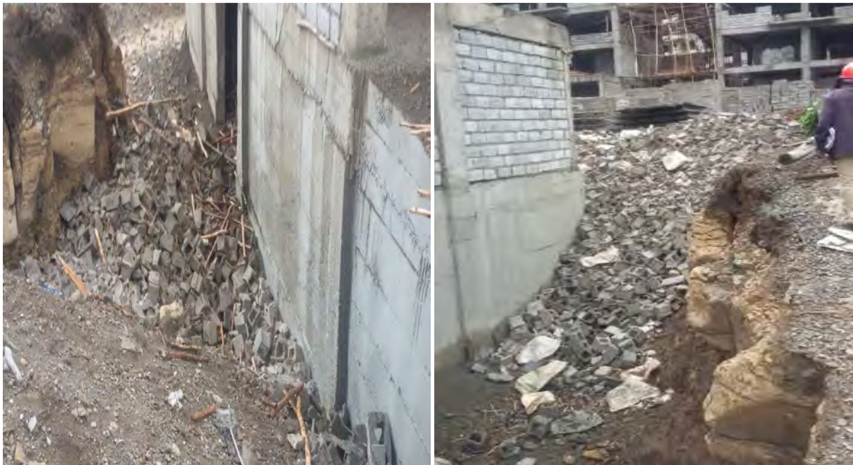
Figure 4.14 Damaged HCB
