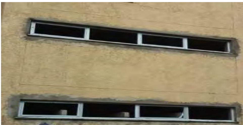
Figure 4.7 Plastering work for covering defect after fixing window frame
