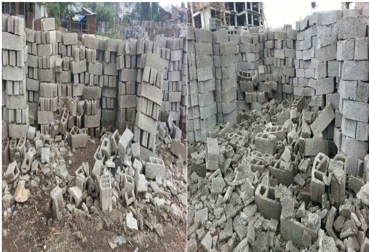
Figure 4.11 Improper storage of HCB
