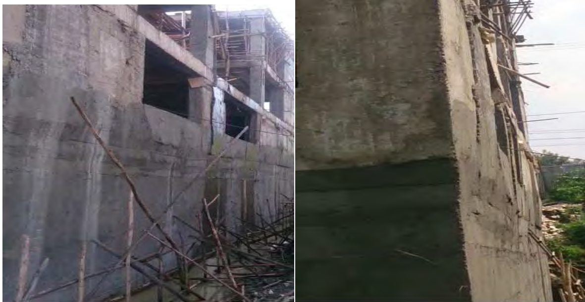
Figure 4.4 Budg shear wall
