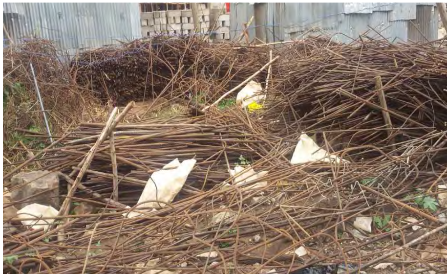
Figure 4.9 Unusable pieces of reinforcement bars
