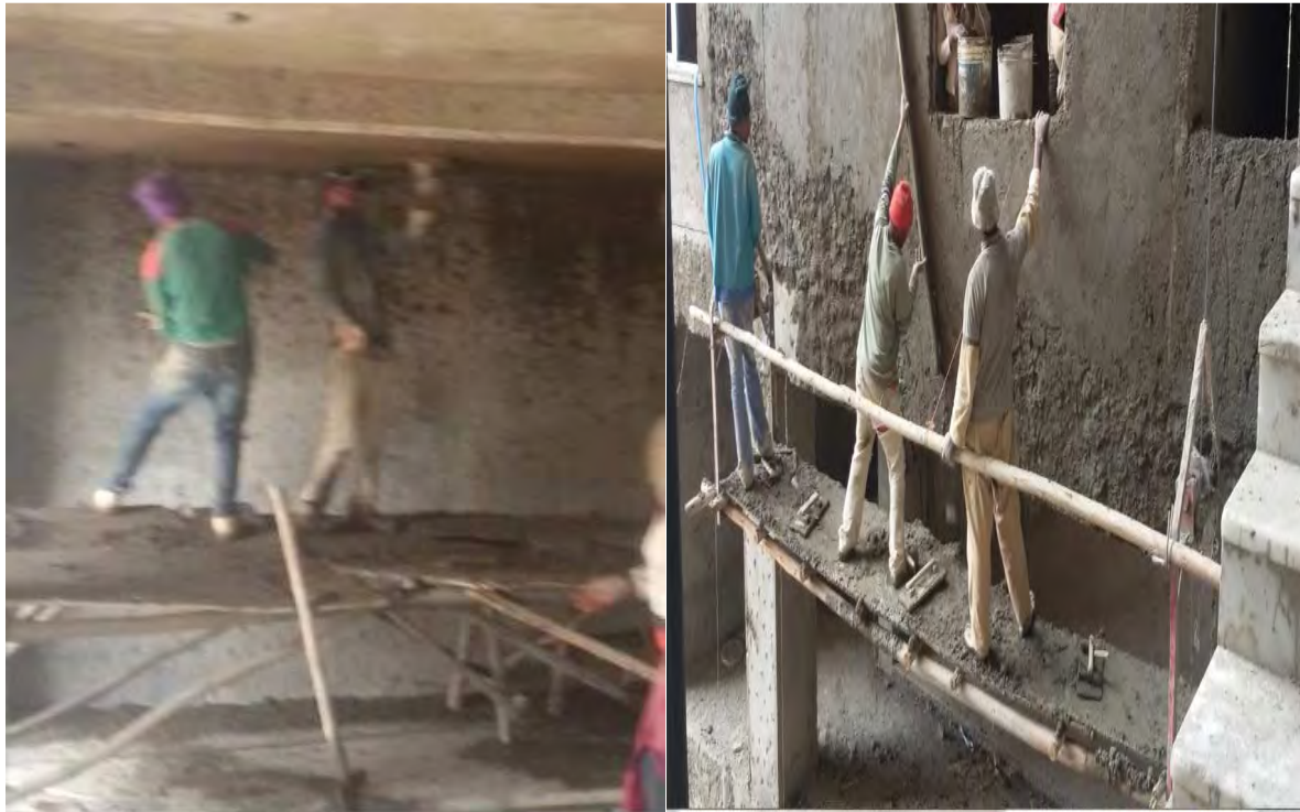
Figure 4.6 Mortar lost during application
