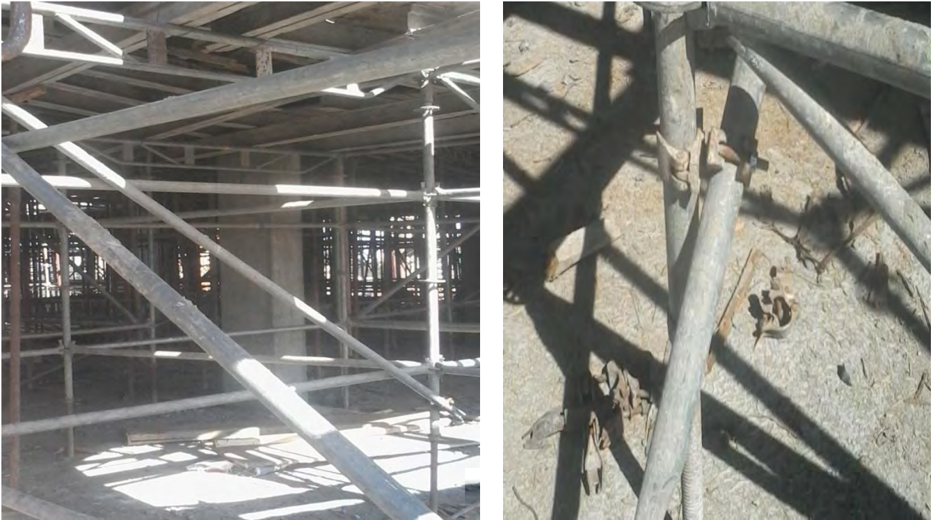
Figure 4.4 Tube and coupler metal shoring
