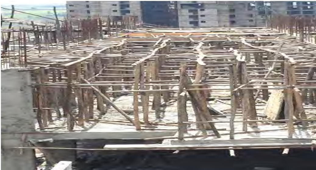
Figure 4.2 Eucalyptus wood shoring for ribbed slab support
