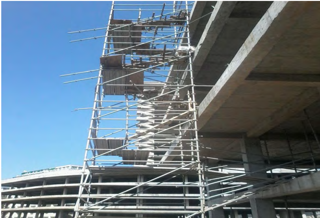
Figure 4.11 Metal scaffolding system around Beherawi theater
