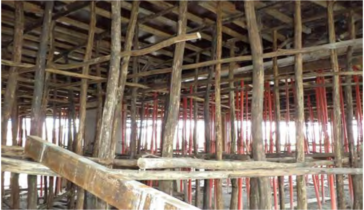
Figure 4.9 Half metal shoring with half eucalyptus wood shoring
