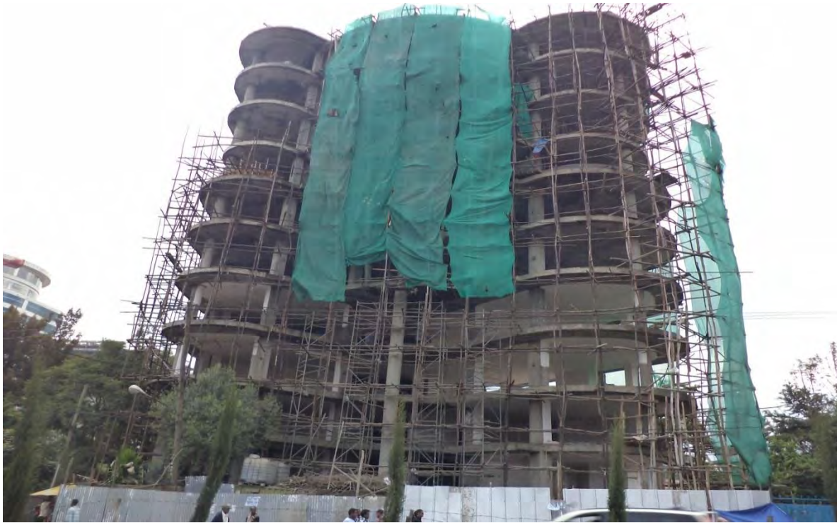
Figure 4.12 Eucalyptus wood metal combination scaffolding system around Kasanchis
