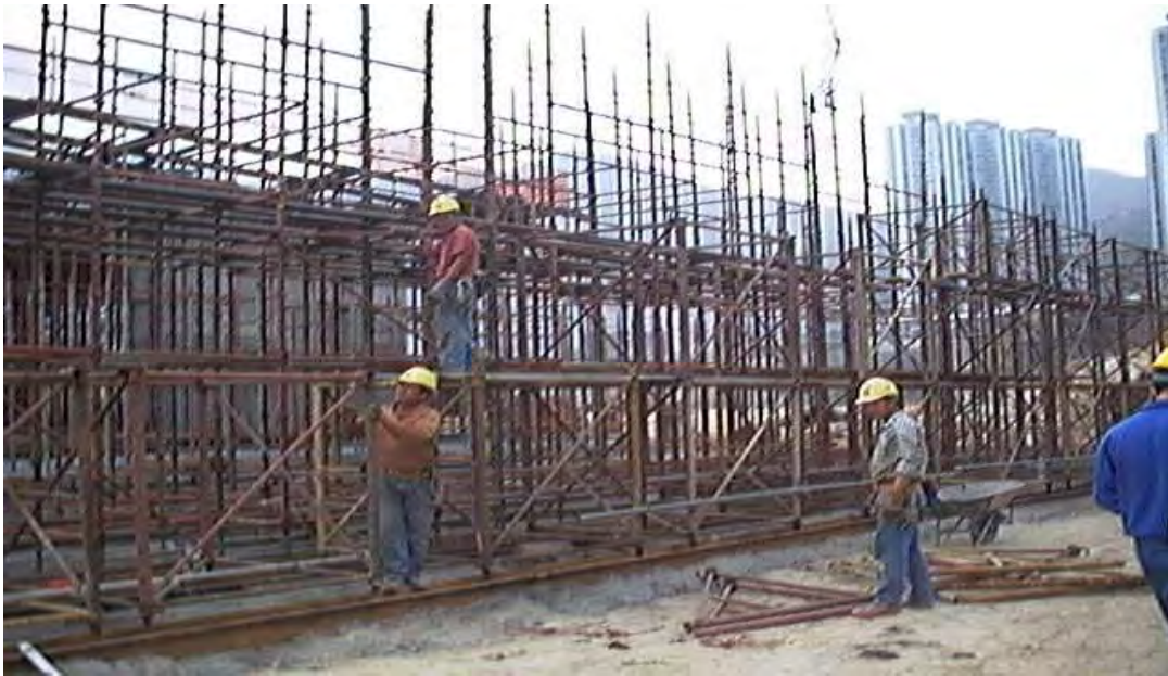
Figure 2.11 Metal Scaffolding Work [22]
