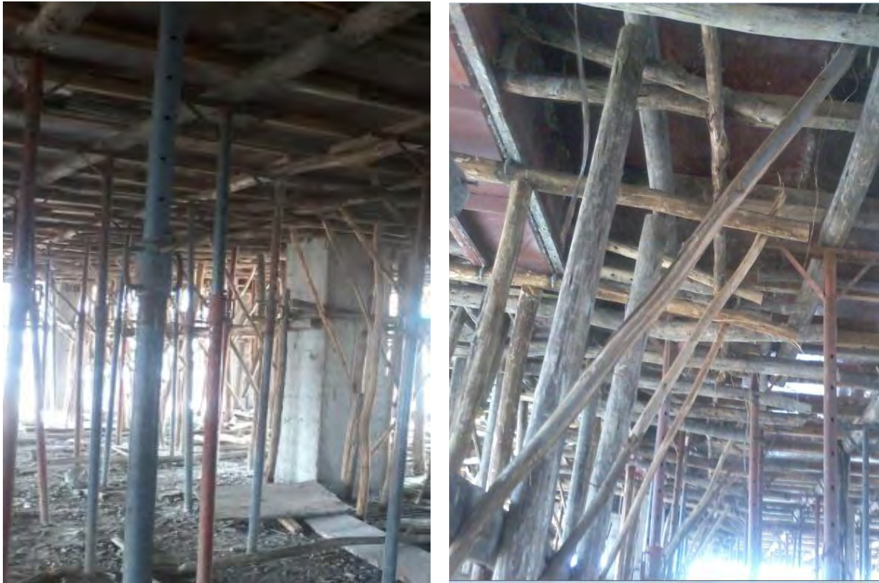
Figure 4.8 Metal shores for slabs and eucalyptus wood shores for exposed beams
