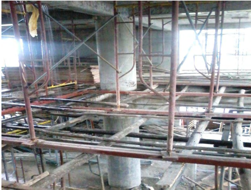
Figure 4.16 Shoring for floor height greater than 8 meters
