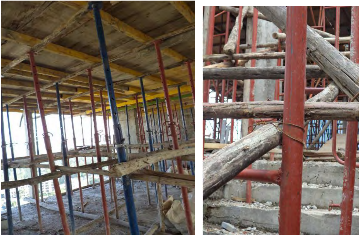
Figure 4.7 Metal frames or tubes with eucalyptus ledgers, transoms and stringers
