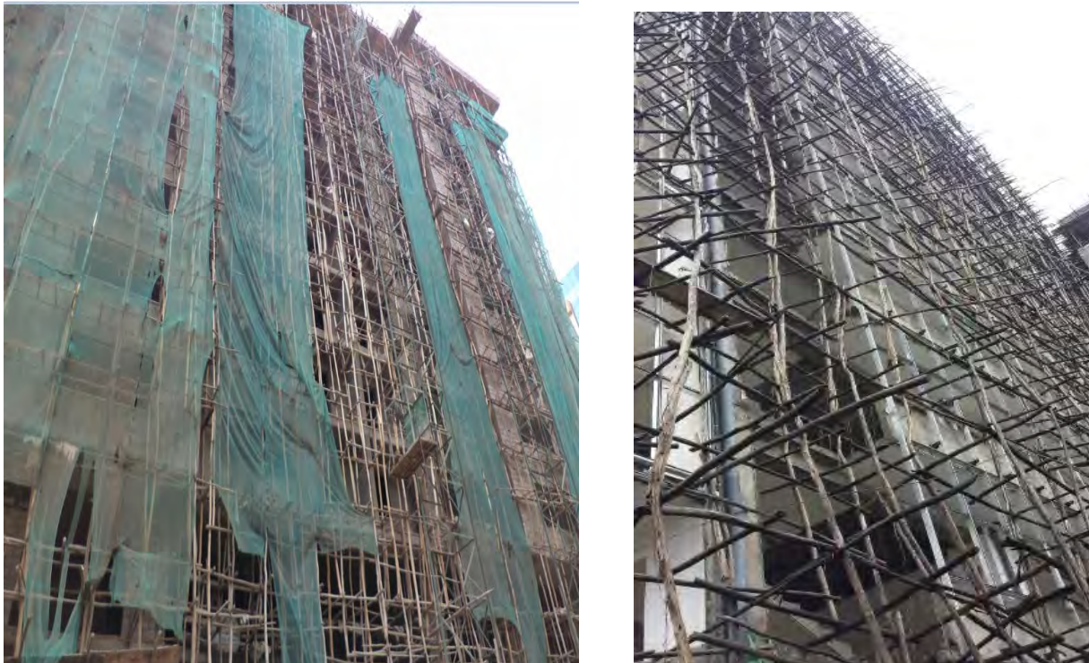
Figure 4.10 Eucalyptus wood scaffolding systems
