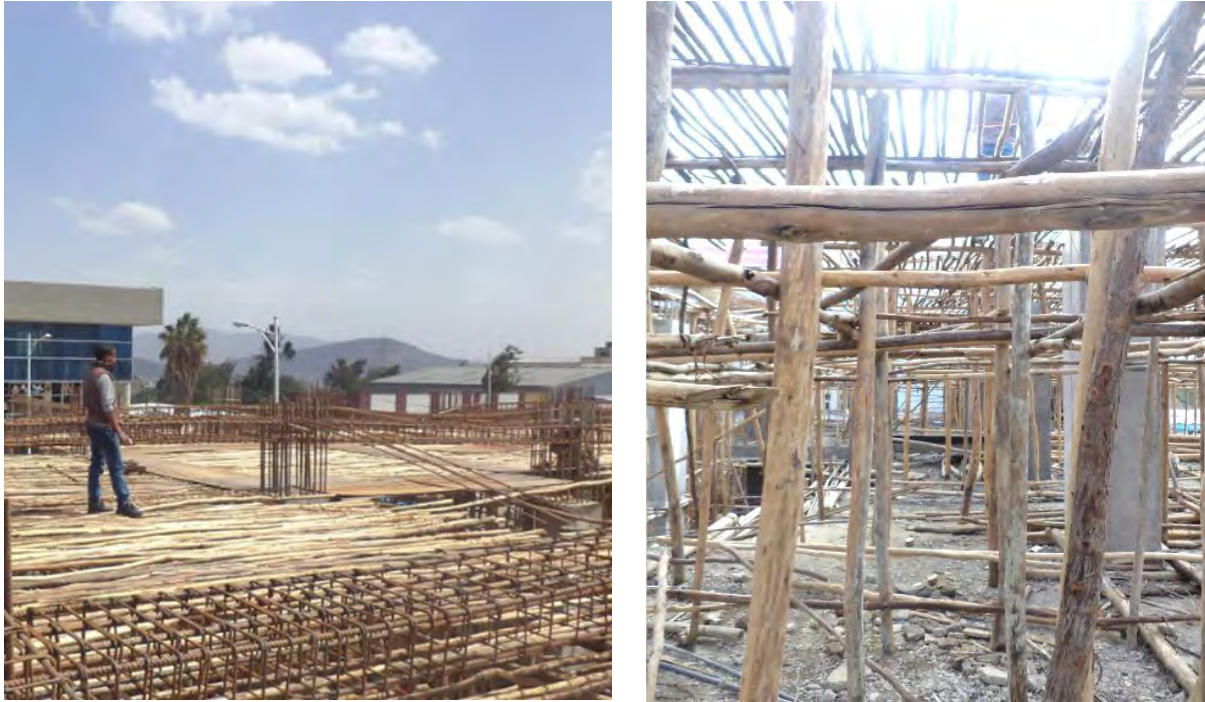
Figure 4.1 Eucalyptus wood shoring for cast in situ slab support
