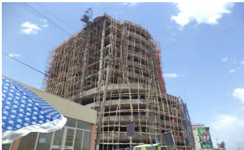
Figure 2.9 Eucalyptus Wood scaffolding in Addis Ababa around 22
