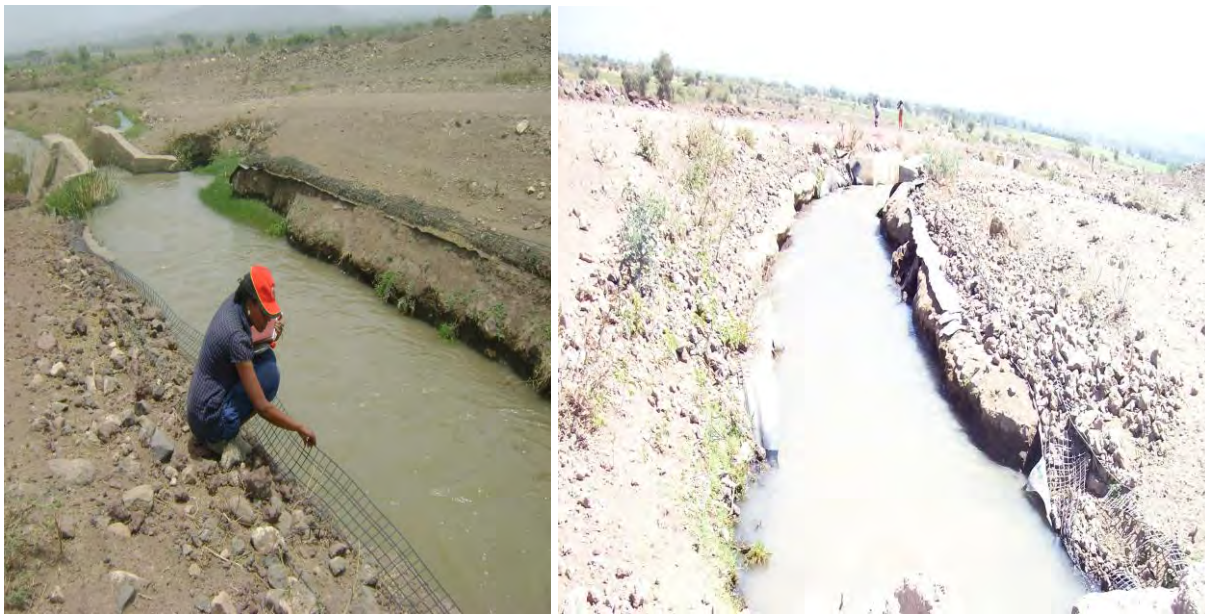
Figure 4.5 Miss use of Geo-membrane
