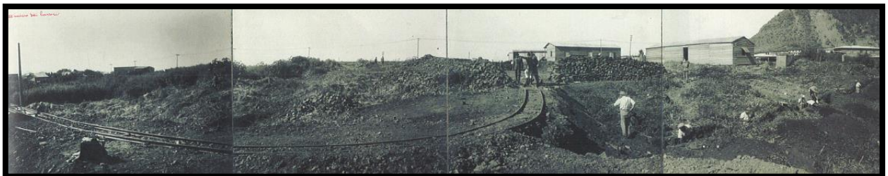
Figure 29: INCIS building site at the beginning of works, Gondar, 1938 (ACS-INCIS).
