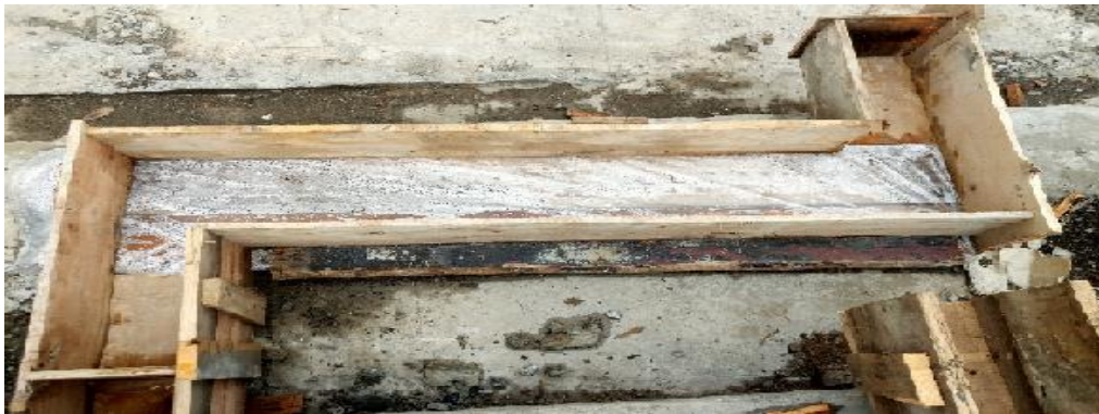
Figure 3-7 plywood formwork preparation
