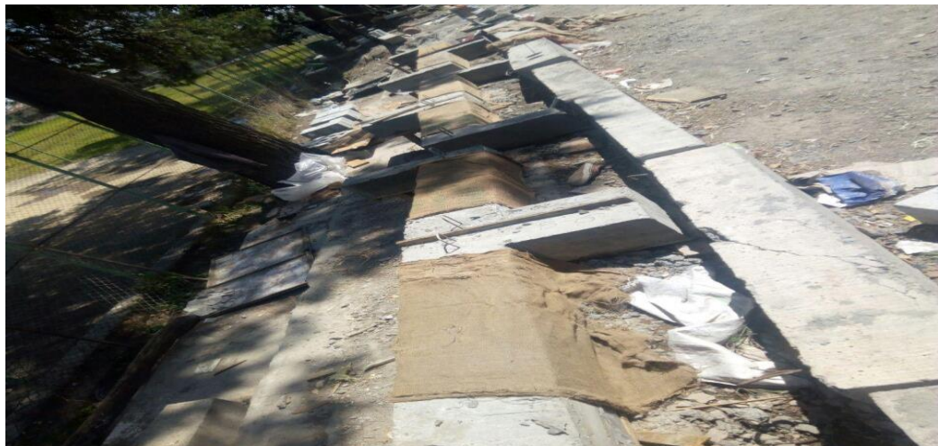
Figure 3-13 curing with covering wet cotton sack
