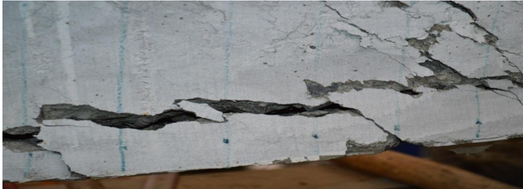
Figure 4-4 post peak cracks of Set-1 specimen 1
