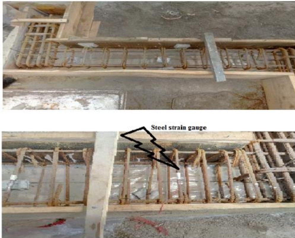
Figure 3-11 Reinforcement cage and formwork of the specimen with attached strain gauge
