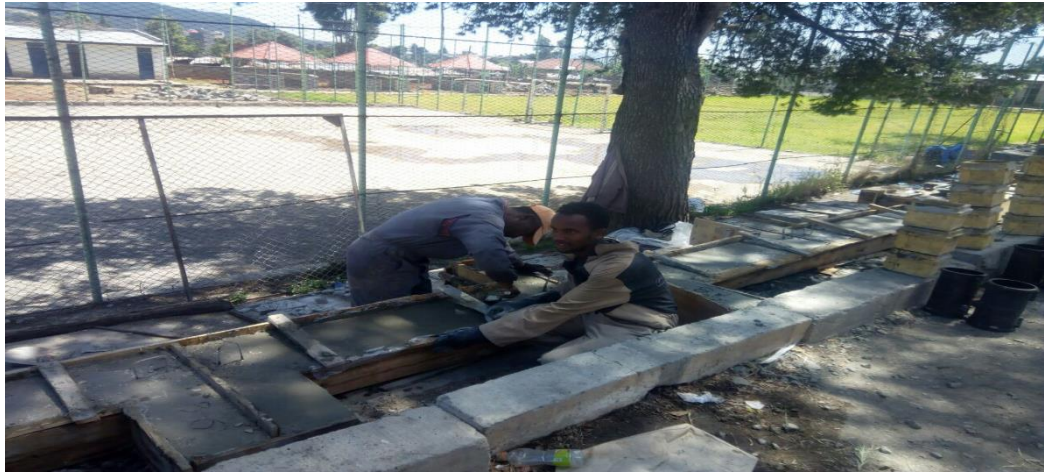
Figure 3-12 Concrete casting outside laboratory
