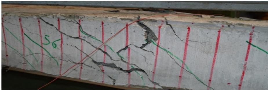
Figure 4-2 NSC_S1_C30 initial to post-peak cracks
