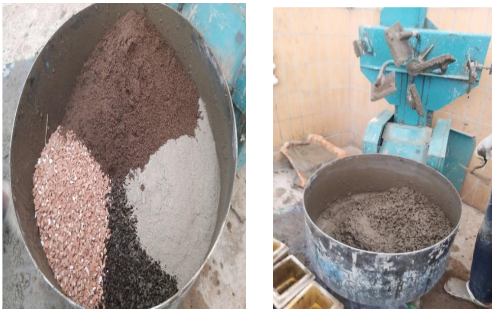
Photo 4. Concrete ingredients before mixed (left) and after mixed (right)
