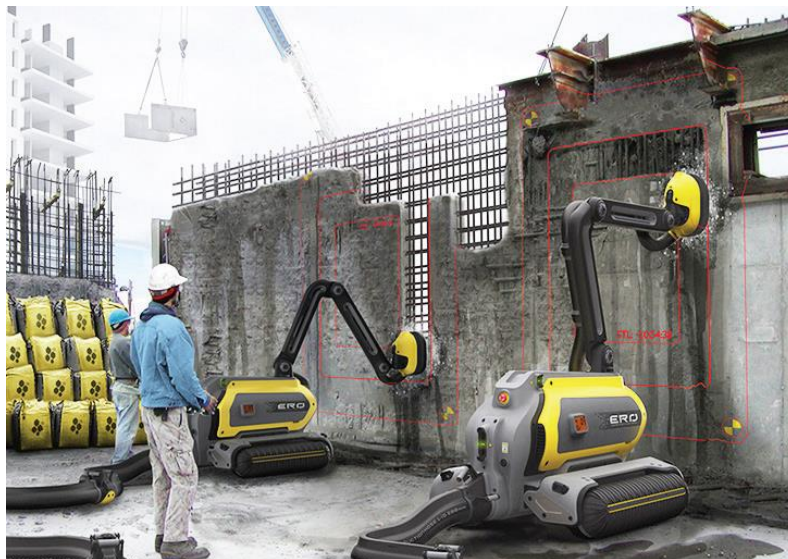
Figure 2-4. Concreting using unmanned machines ( https://roboticsbiz.com/different-types-of-robots-transforming-the-construction-industry/ )
