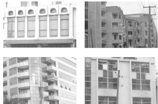
31. Some the building details in CHAGS area
