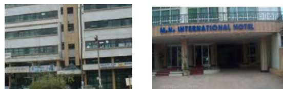
25. Some of the buildings with visible entrances CHAGS area
