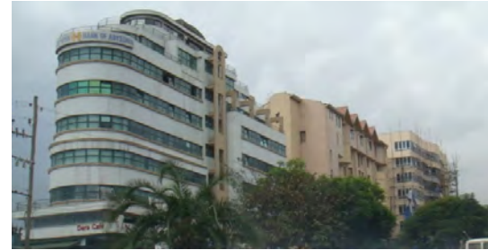
28. Some of buildings in good scale and skyline in CHAGS area
