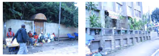
66. Some of the blank walls as detractors in LRS-BT area
