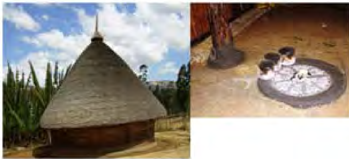
Figure 10: Typical tukul in Butajira and interior floor with traditional stove and axis pole at the center
