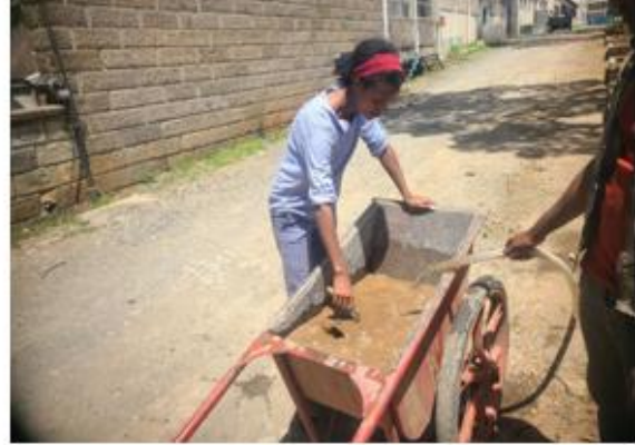
Photo: purchasing and washing sand and aggregate
