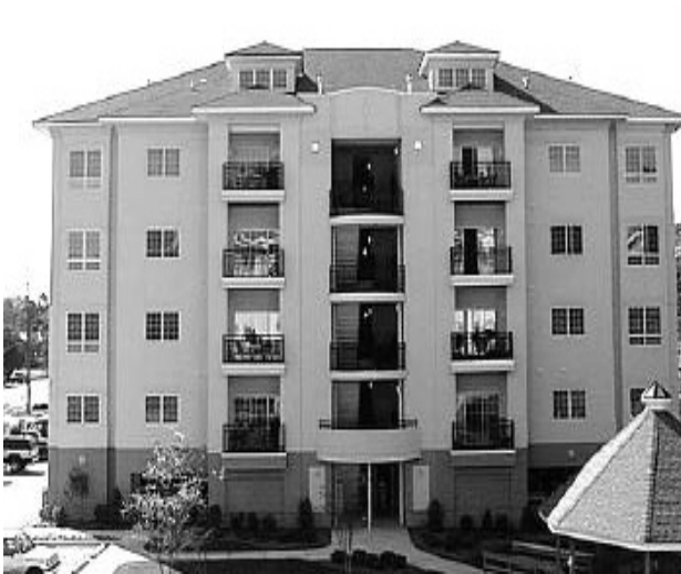
Picture.2.3. Open Stairwells and Stair Landings are easily visible. Source: General Guidelines for Designing Safer Communities
