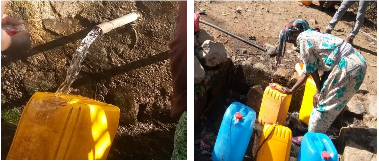
Plate 4: Developed springs having a yield of 1L/s (left) and 0.5L/s (right) which emerged in the Ashange basalt to the north of Hayk towns, these springs have low TDS, EC, and temperature and they are used as drinking water for the local community.
