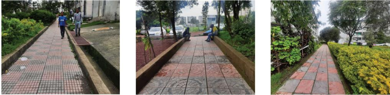
Figure 11: Sidewalks (Source: Picture taken by the Researcher, 2022)
