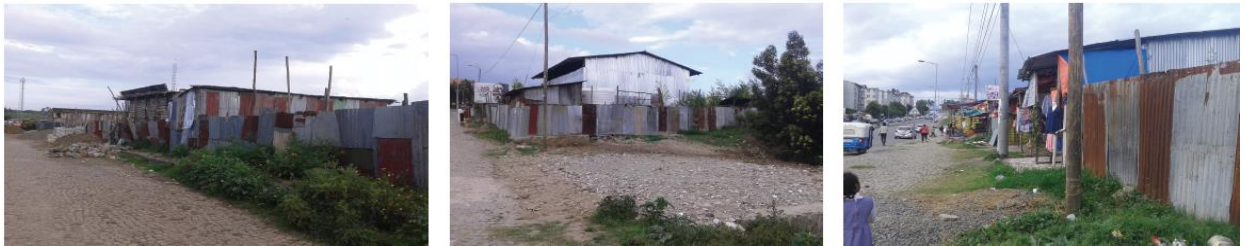
Figure 6: Open Spaces converted to built-up area (Source: Picture taken by the Researcher, 2022)
