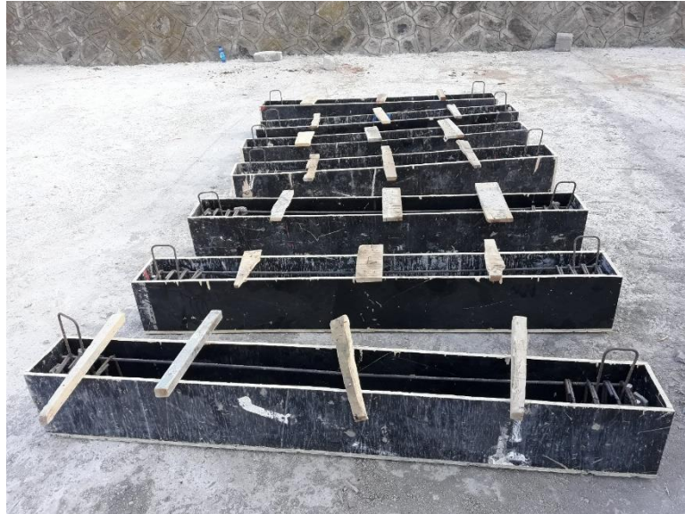
Figure 3.5: Formwork
