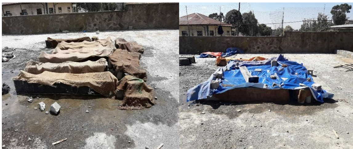
Figure 3.6: Curing of casted specimen
