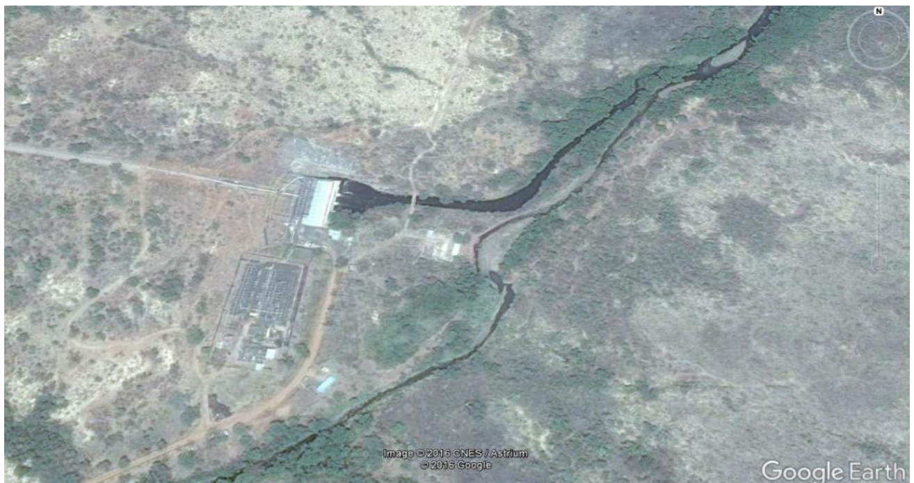
Figure 4-30: Fincha'a Hydroelectric Power House downstream of the fall
