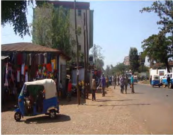
Jemila G+3 building situated to about 4.2metres (3m on the ground & 1.2m extended cantilever above first floor) on the public road sides of way.
