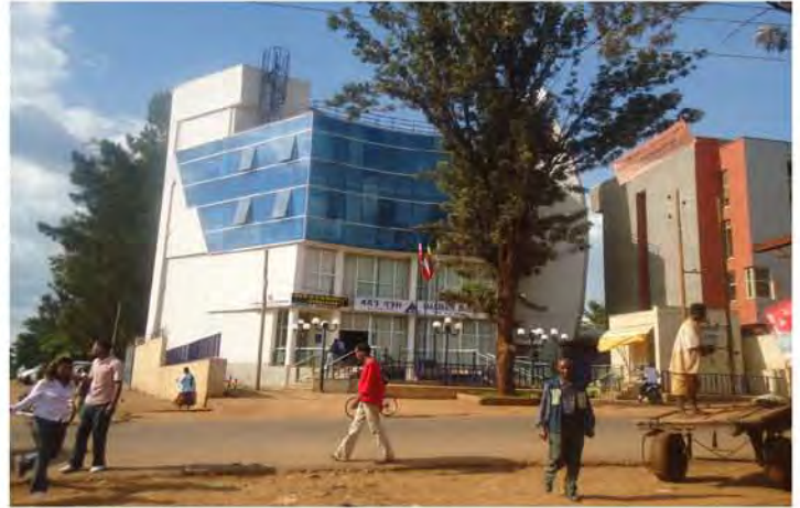
Dashen bank G+3 building situated to about 1.2metres from west side on the public road sides of way.
