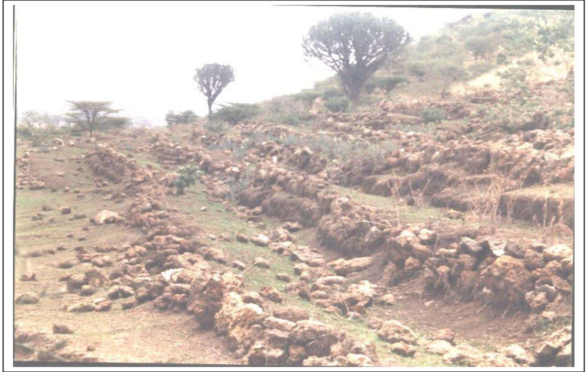
Figure 1. Hillside terraces that lack maintenance work
