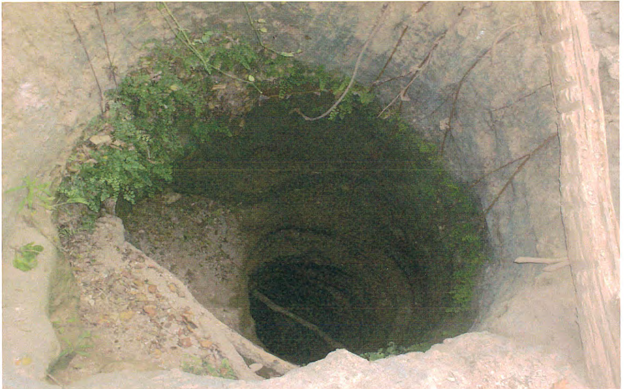
Figure 10. Deep wells ( Tulla ) estimated to 30 meter depth
