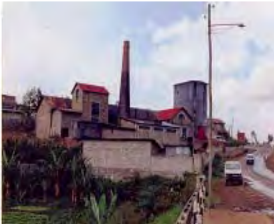
Figure 1. Vegetables farm beside Addis Ababa Winery irrigated with water contaminated with the effluent (Photo EPA, 1997).
