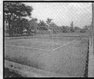
Ground Tennis field under construction
