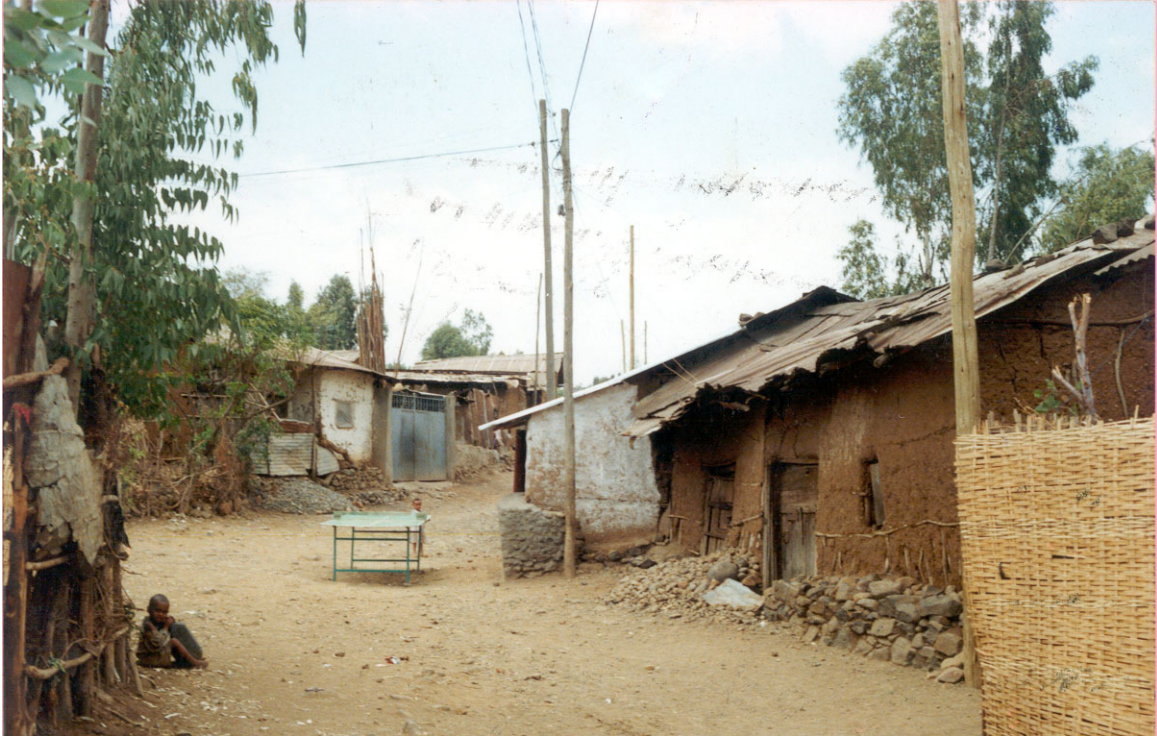
Fig. 4.3: Aspects of Most Housing Units in Gondar Town.
