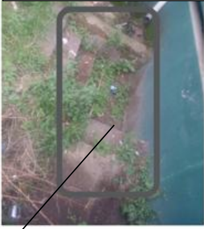
Location – right courtyard stair
