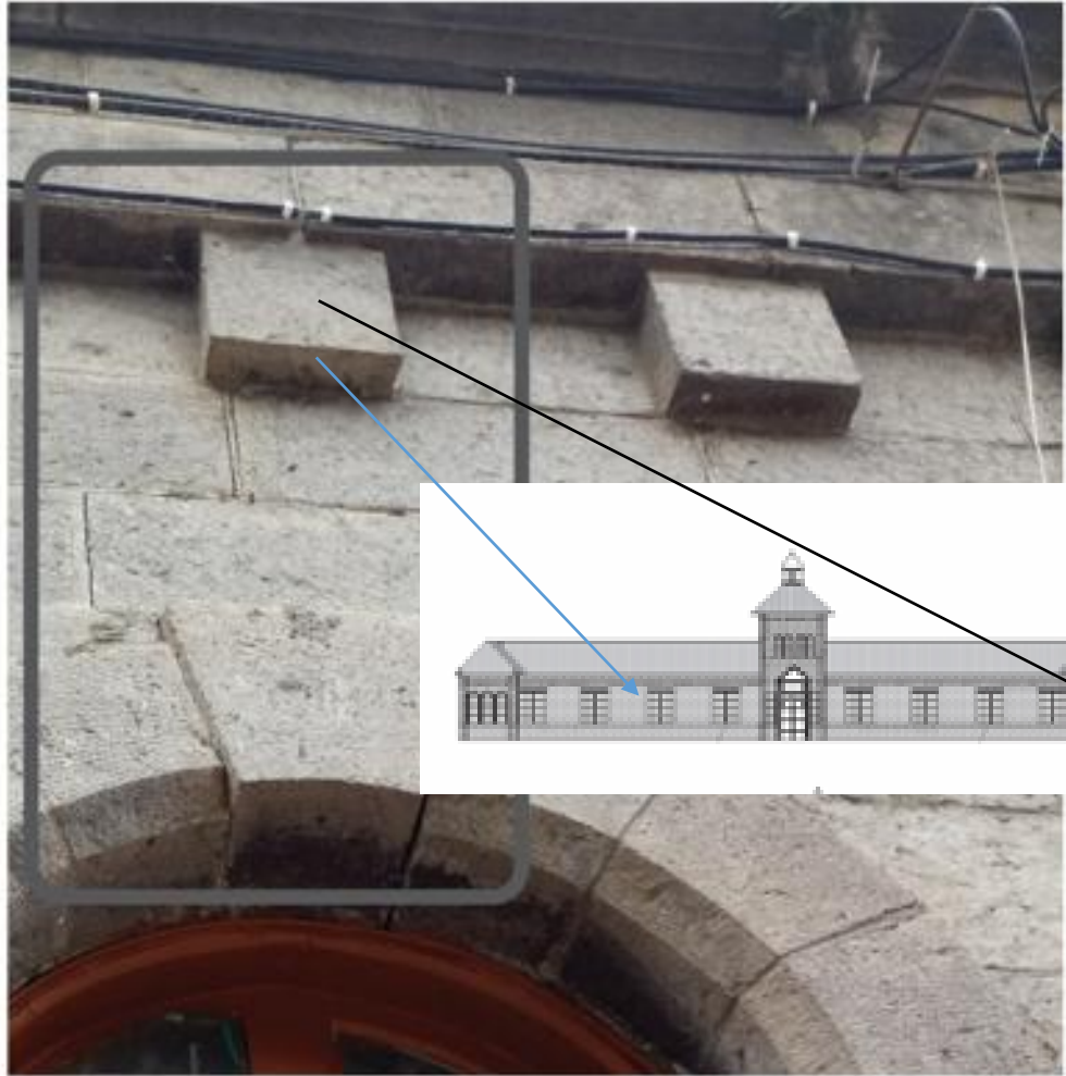
Location – right side –front elevation – above arched window
