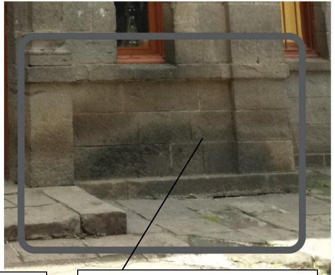
Location – front side on the wall
