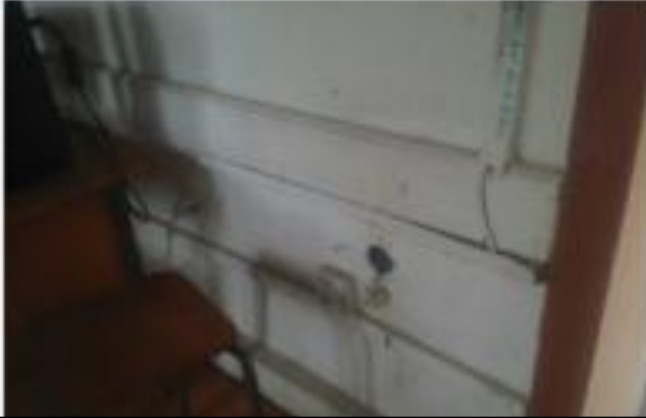
Location – inside the semi basement rooms
