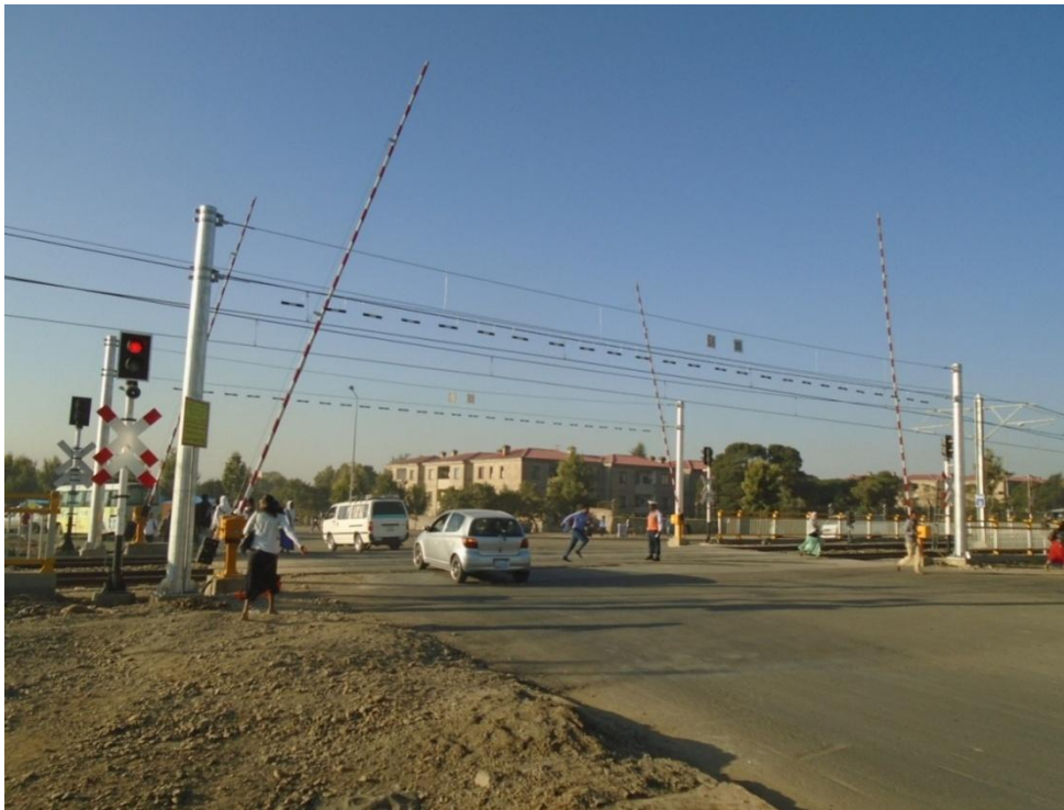
Figure 1-2 AA-LRT level crossing signaling around CMC area
