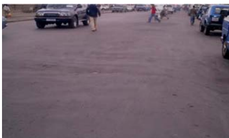
Figure2.7 Corrugations from site survey & severity level as per (GTC, 1998)
