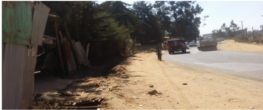
Figure 4.4 Proper drainage problems
