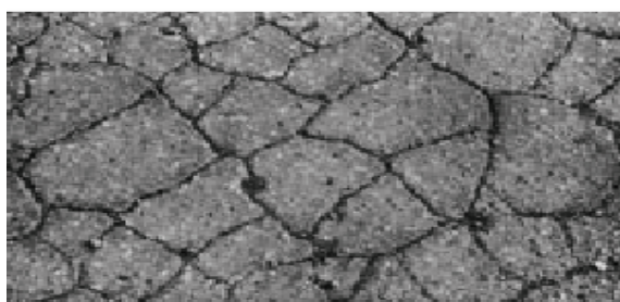
Figure 2.3 Alligator cracking from site survey & severity level as per (GTC, 1998)
