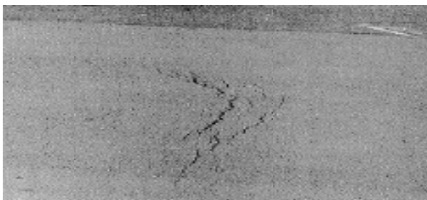
Figure 2.18 Slippage cracks
