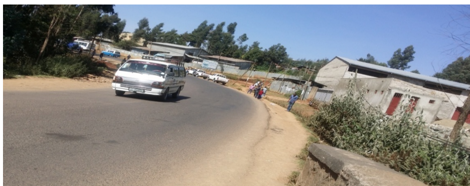
Figure 4.3 Few crossing structures of existing Culvert
