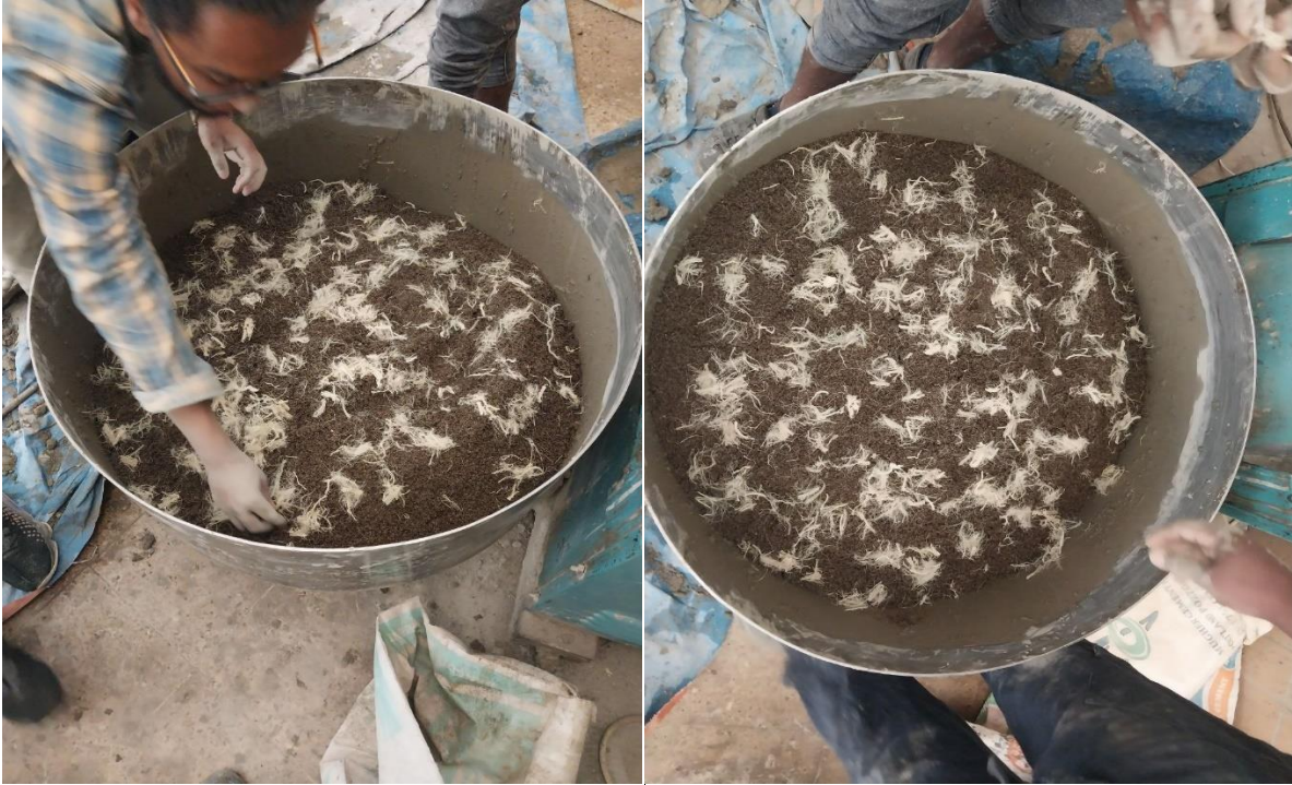
Figure 3.8: PALF with concrete in mixer
