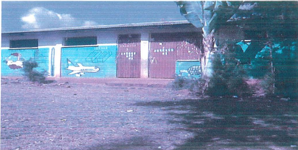
Figure 1: Primary School of Addis Alem Kebele
