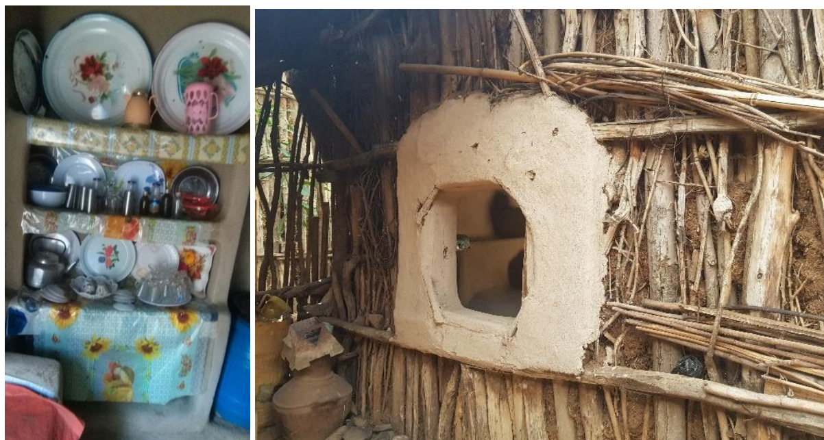
Figure A.17 W/ro Melkenesh Ahmed fuel-saving stove chimney exit for smoke
